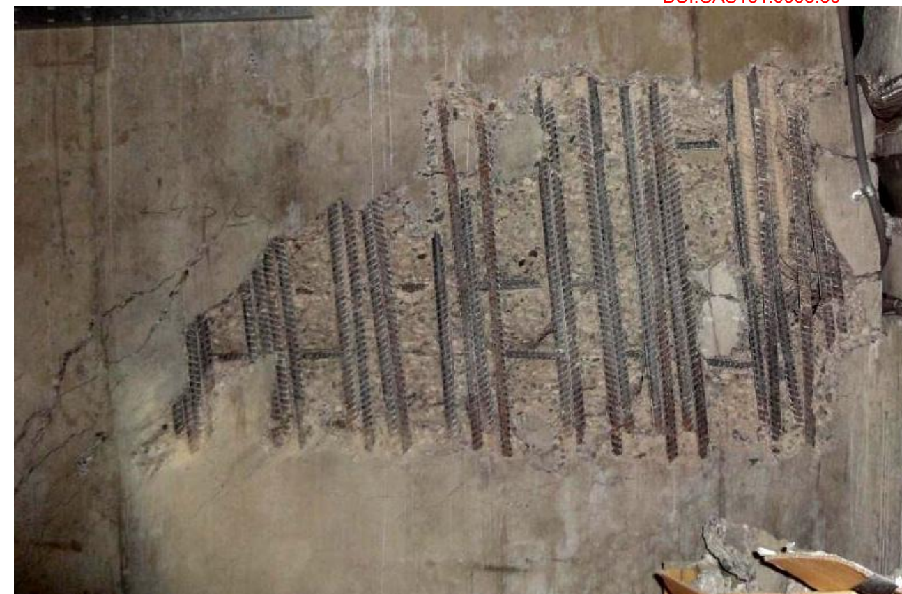
Photo 15 - Near-lap failure grid 8 cantilever transfer beam
