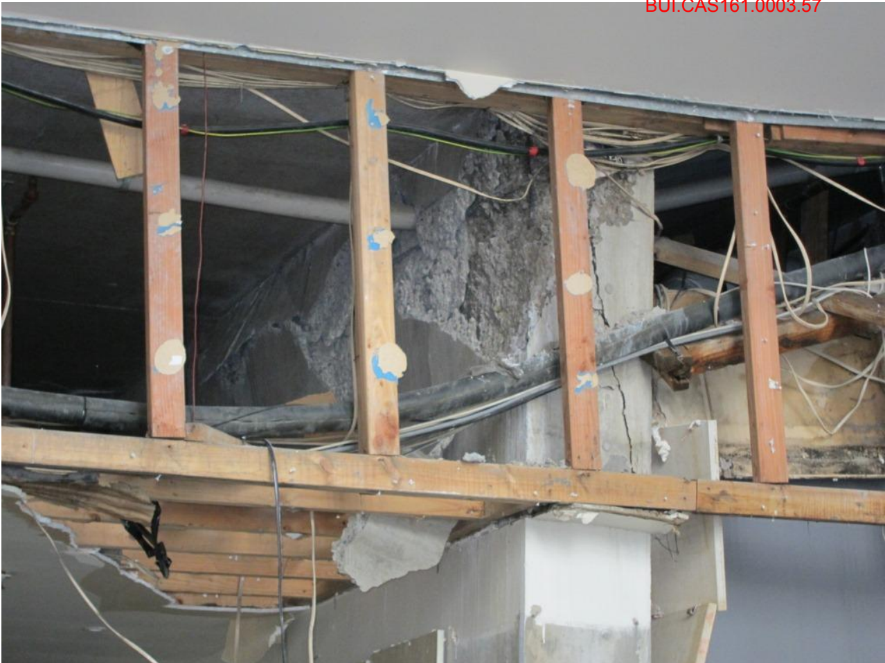
Photo 7 - Shearwall D5-6 - Hinging at top of ground floor
