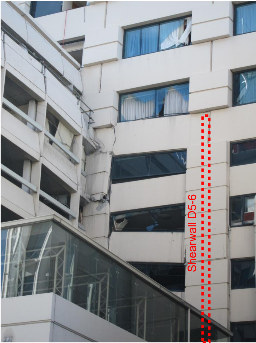
Photo 5 - Damage at junction between podium and tower - not related to pounding
