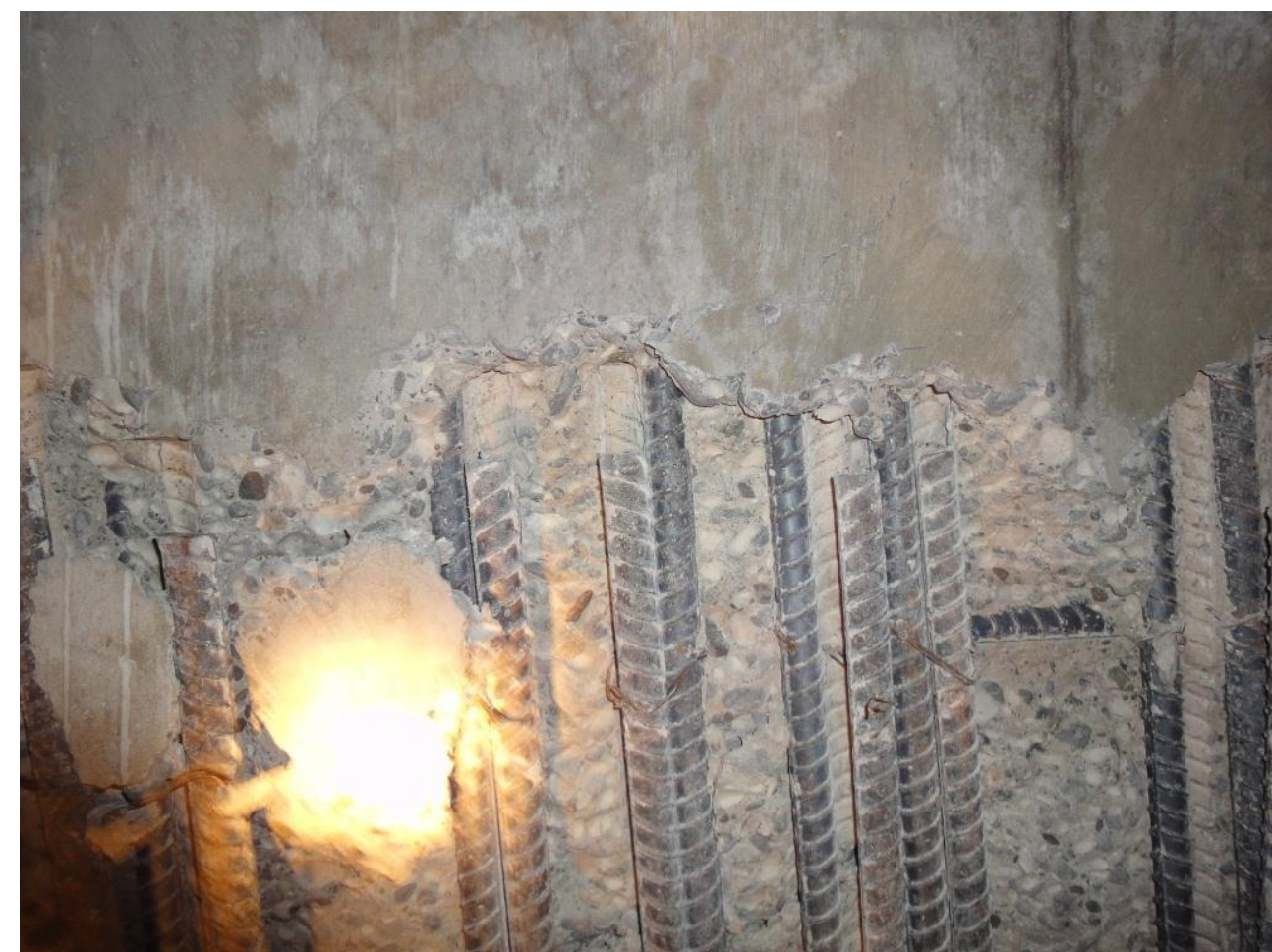
Photo 16 - Near-lap failure grid 8 cantilever transfer beam
