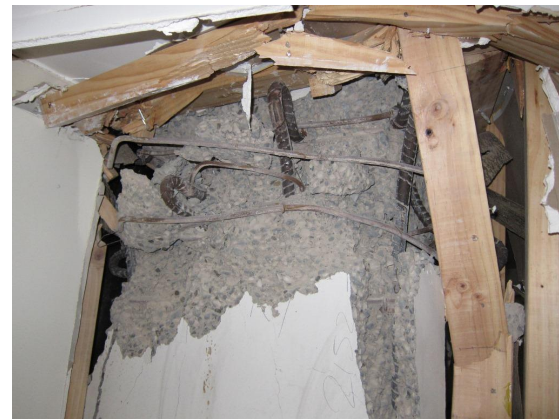
Photo 22 - Crushed columns at level 10, lines 5 & 6
