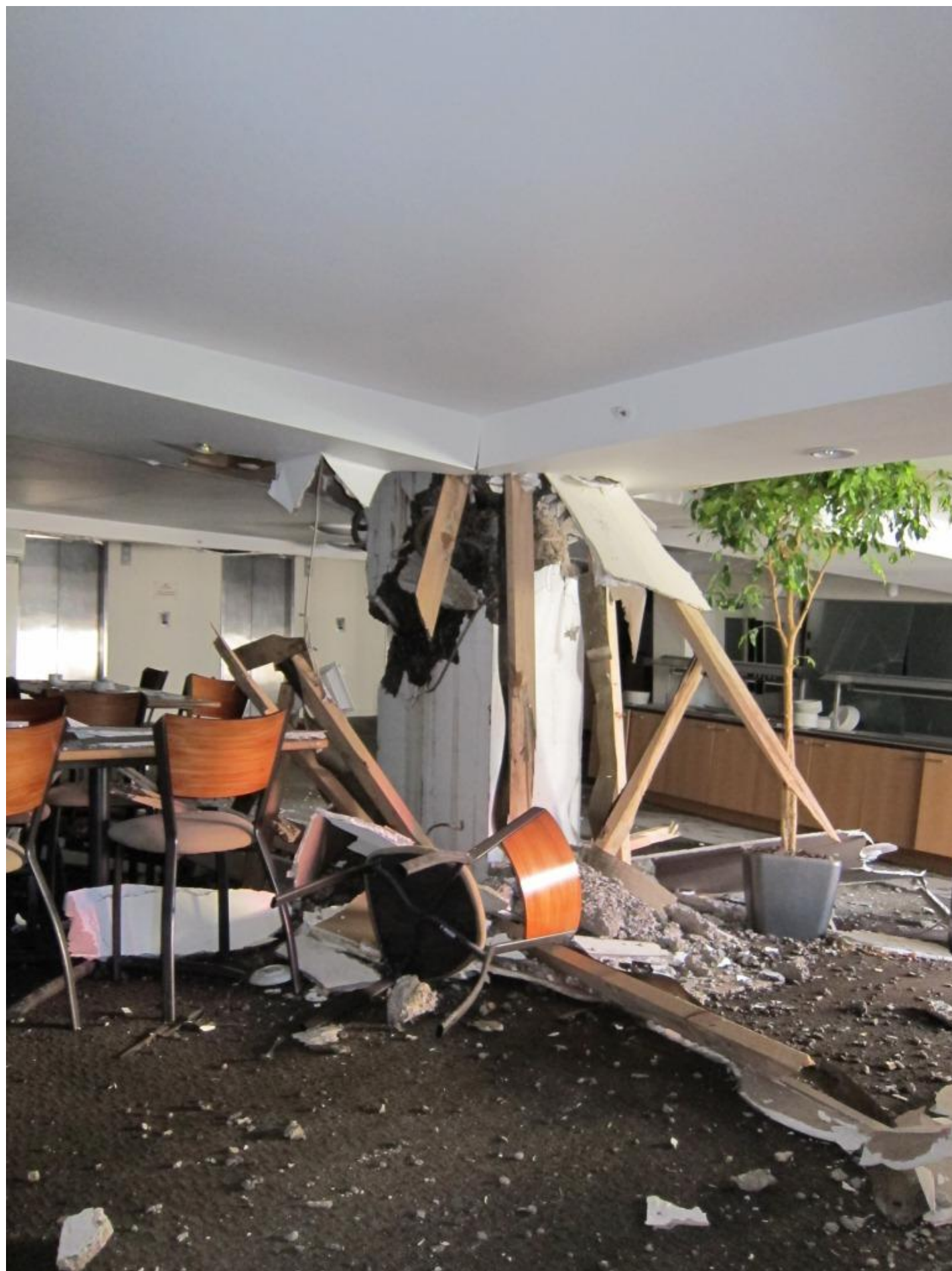
Photo 20 - Crushed columns at level 10, lines 5 & 6
