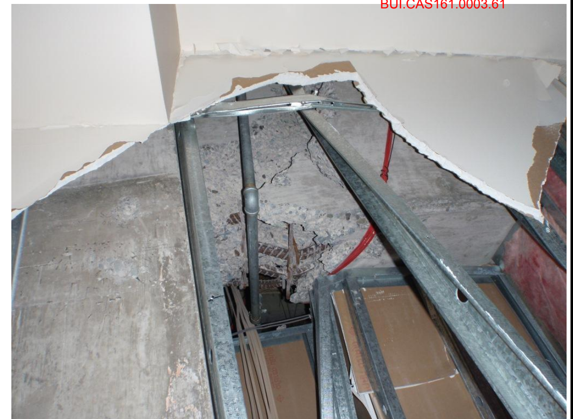
Photo 18 - Hingeing in grid D tower beams
