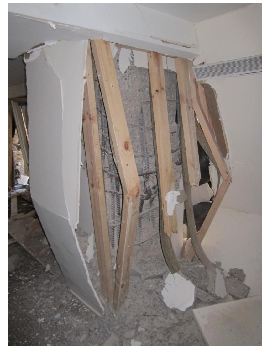
Photo 21 - Crushed columns at level 10, lines 5 & 6
