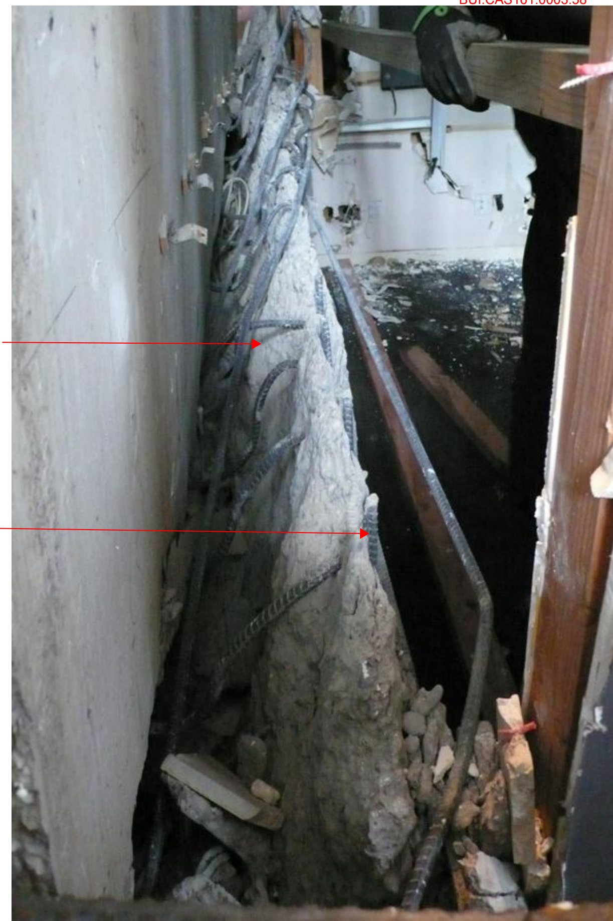
Photo 10 - Shearwall D5-6 Failure - Close-up
