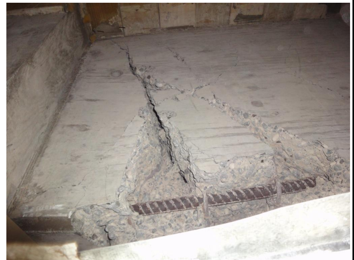
Photo 19 - Hingeing in grid D tower beams
