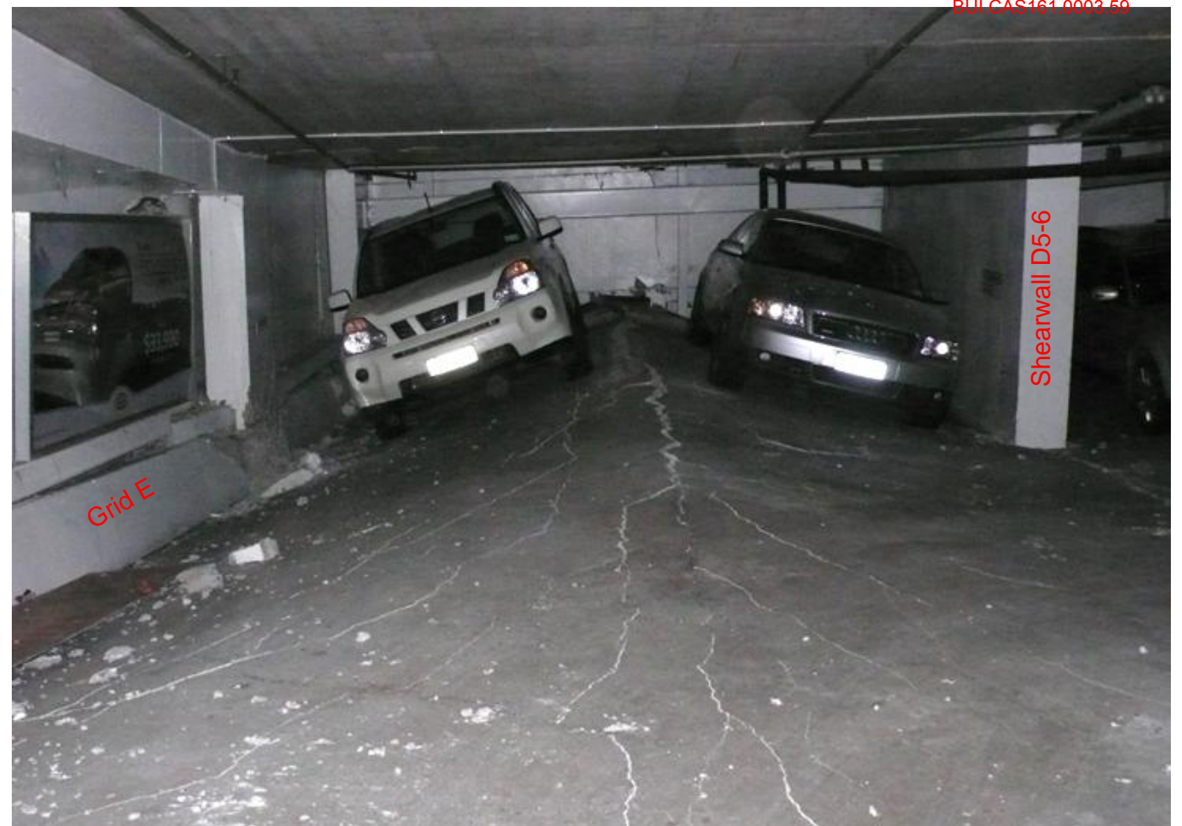
Photo 13 - Folded slab at level 2
