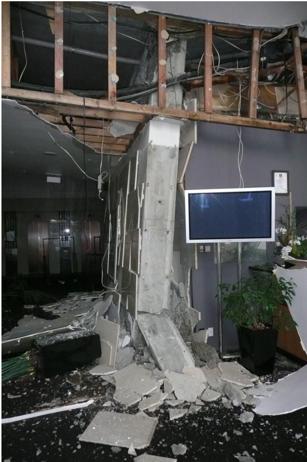
Photo 6 - Shearwall D5-6 - Base Failure
