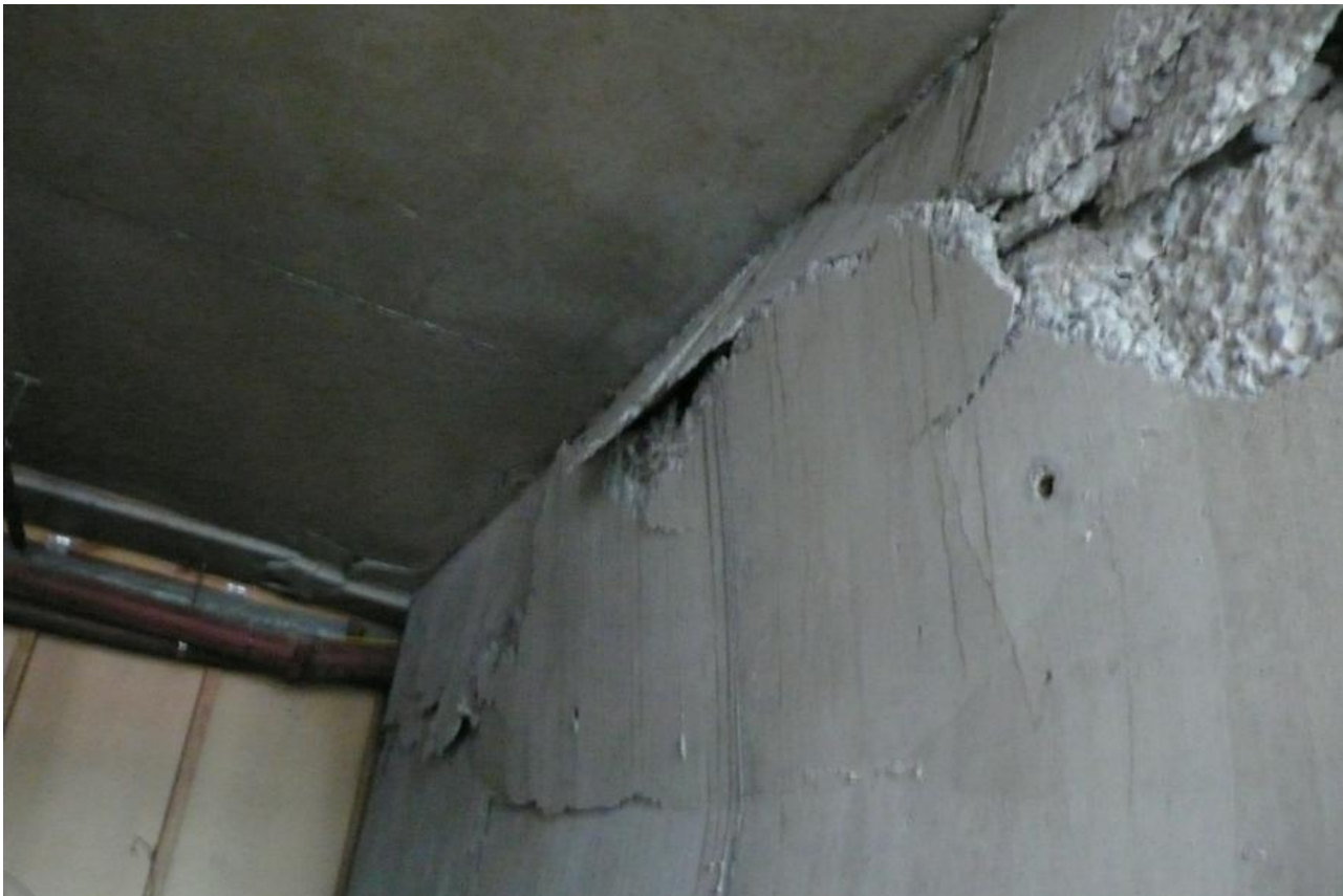
Photo 8 - Shearwall D5-6 - Hinging at top of ground floor
