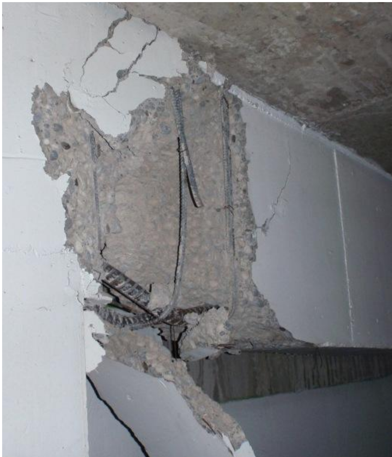
Photo 14 - Hingeing in grid E beams 6-7
