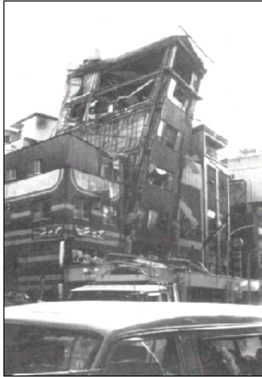
Figure 8.2: Slender concentrically braced framed building with failure of brace to frame connections, Kobe earthquake
