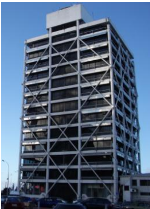
Figure 5.11. Union House, Auckland, base isolated using flexible piles and energy dissipaters.
