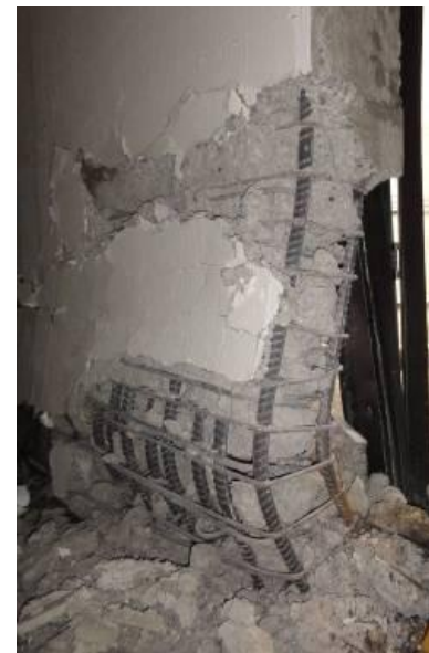
(b) Severe damage to reinforced concrete wall, with local buckling at the toe of the wall.
