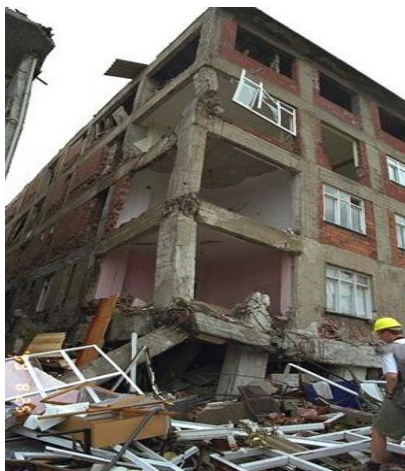
Reinforced concrete building with masonry infill (Turkey, 1999)
