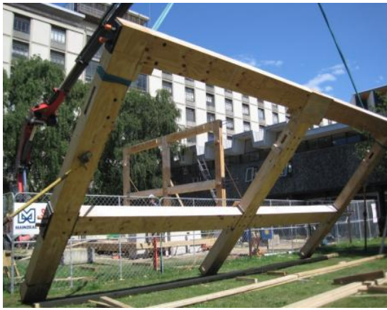
(a) Post-tensioned frame being erected.
