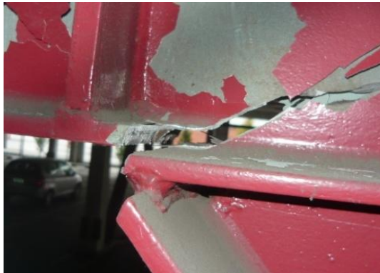
Figure 4.7. Fracture in steel frame near welded connection.
