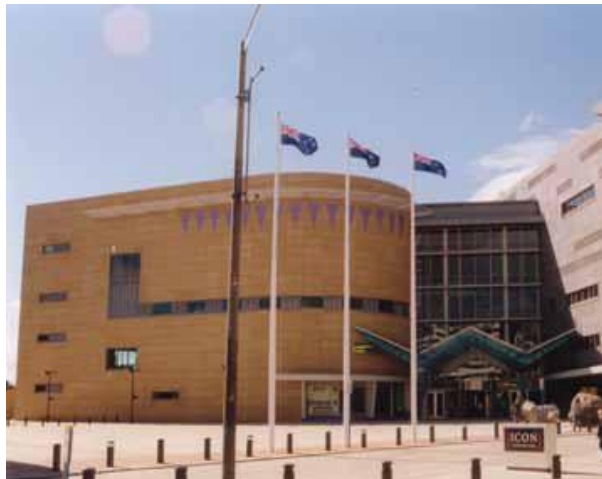
Figure 5.13. Te Papa Museum in Wellington has base isolation with lead rubber bearing (Skinner et al., 2000).
