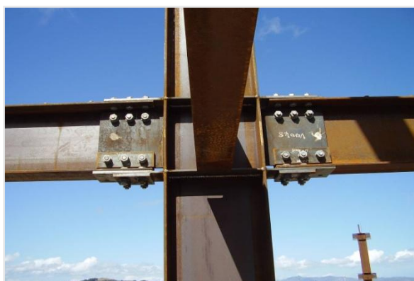
(a) Sliding hinge AFC
