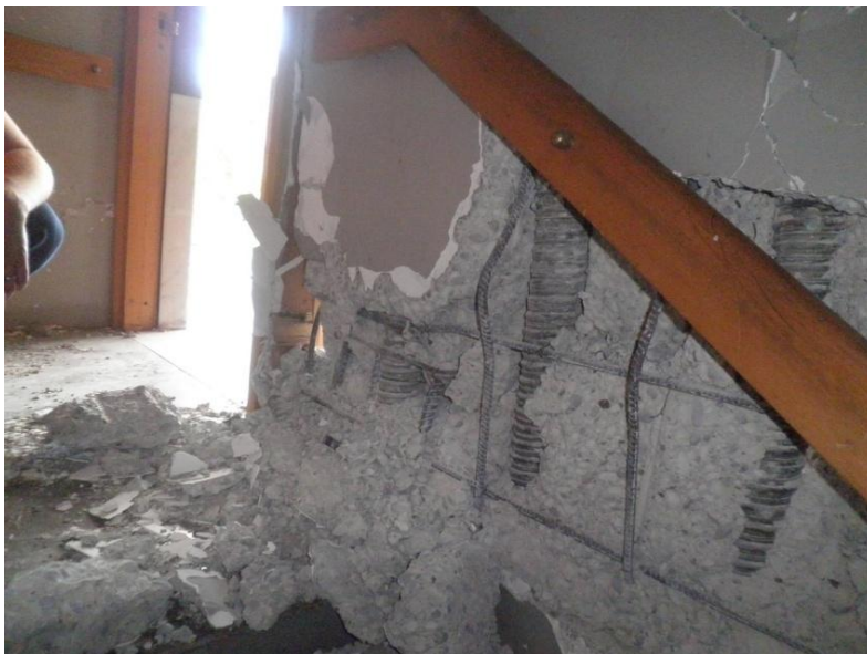
(a) The system for joining precast concrete wall panels fails through insufficient confining reinforcement.
