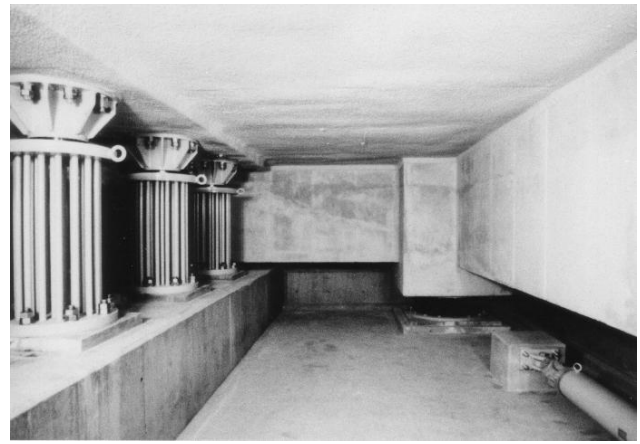
High damping rubber bearing, steel dampers and oil damper in basement of Bridgestone Toranomon Building, Tokyo.
