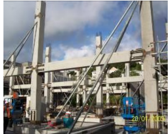
Figure 7.14. First multi-storey PRESSS-Building in New Zealand (Cattanach and Pampanin, 2008).
