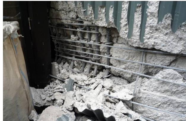
(b) Severely damaged end of structural wall.
