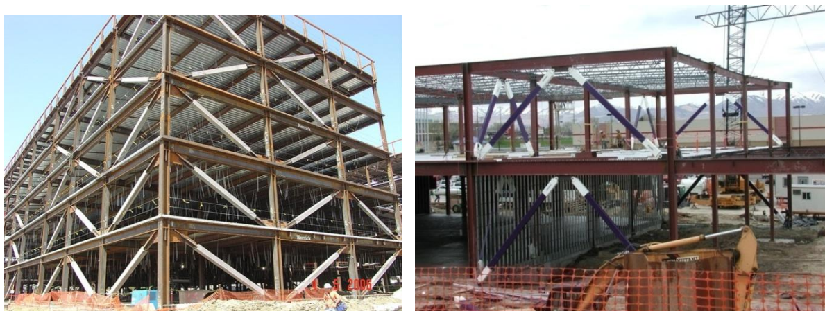
Figure 8.11. Diagonal and inverted V-braced BRB concentrically braced frame structures (AISC, 2007).
