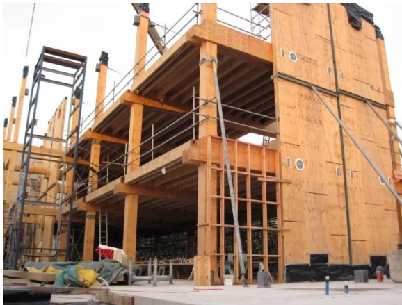
(a) The building under construction. Post-tensioned walls to the right.
