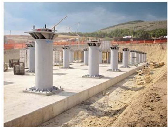
(b) Base isolators on steel columns
