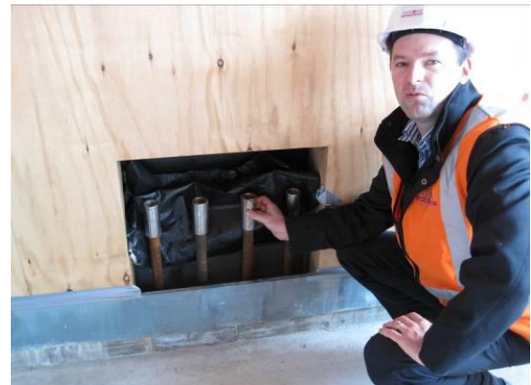
(d) Threaded couplers for Macalloy bars at base of wall.
