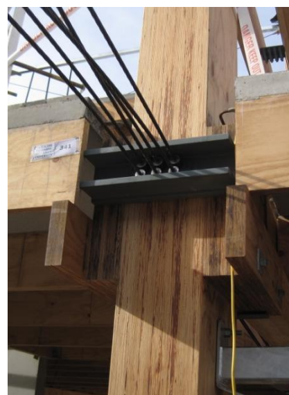
(b) Detail of post-tensioned anchorage
