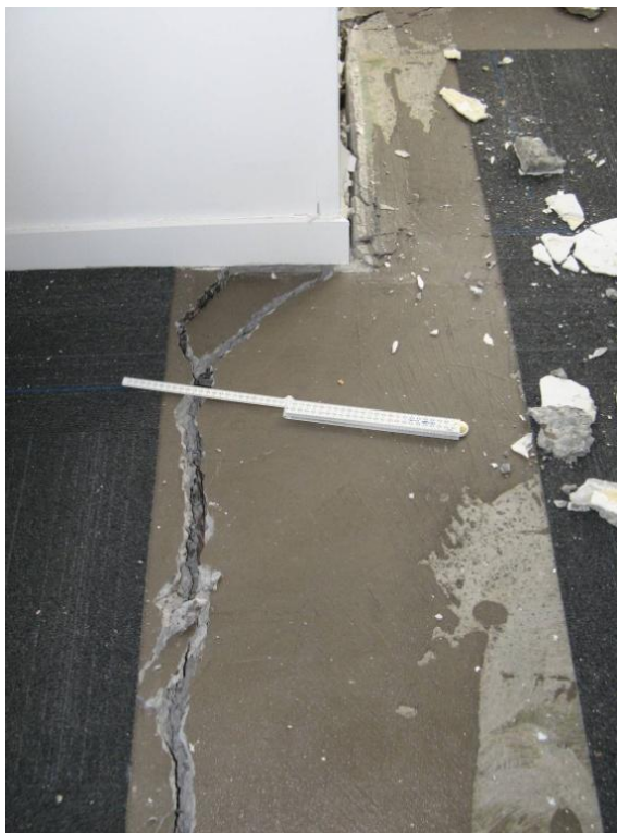
(a) Frame has elongated and moved away from the precast concrete floor
