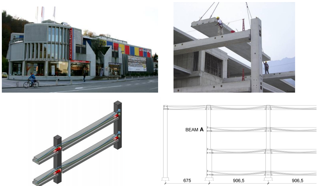
Figure 7.13. Photographs and sketches of the post-tensioned “Brooklyn System” (Pampanin et al., 2004).
