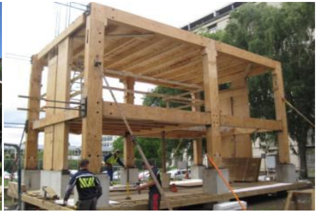
(b) Structural framework in place.
