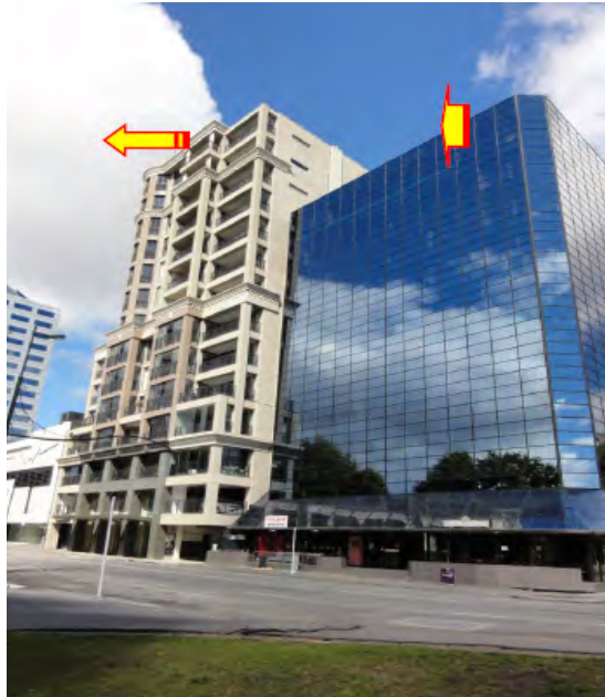
Figure 18. Residual tilts of adjacent buildings
