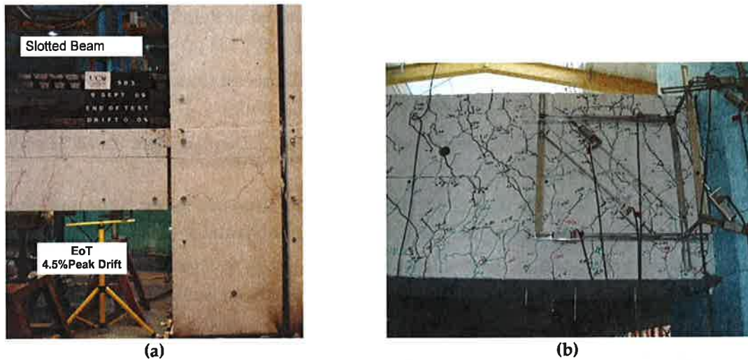
Figure 6.10. (a) Slotted reinforced concrete beam after 4.5% peak drift (Au, 2010). (b) Damage to conventional beam after 3.0% peak drift (Lindsay, 2004).
