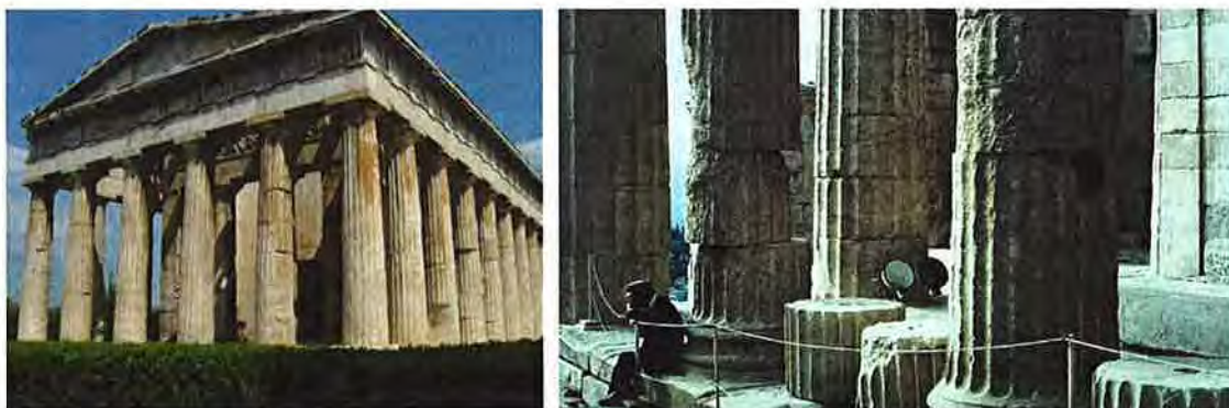
Figure 6.3. Earlier implementation of a self-centering limited-damage rocking system, for earthquake loading (Dionysus temple in Athens).
