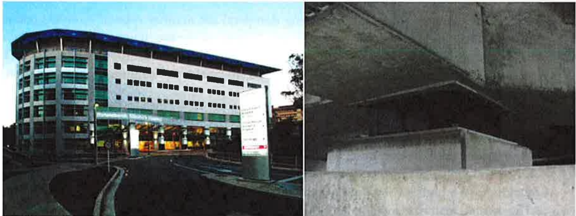
Figure 5.10. Christchurch Women's Hospital, showing one of 40 lead-rubber bearings.
