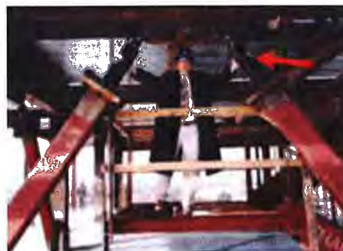
Figure 5.6. Application of fluid viscous damper. http://www.wbdg.org/resources/seismic_design.php
