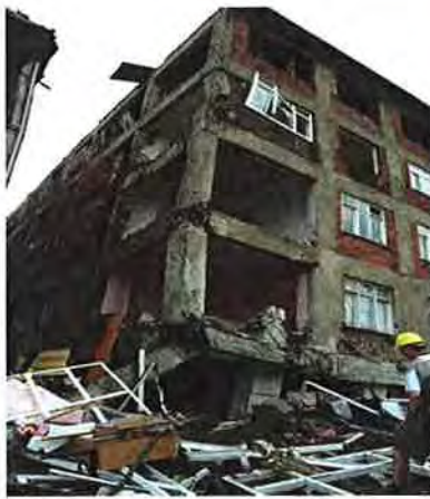
Reinforced concrete building with masonry infill (Turkey, 1999)
