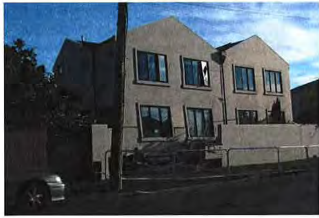
Three-storey apartment building which collapsed to two storeys (Christchurch 2011)
