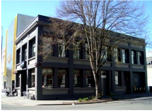
(a) Exterior view
