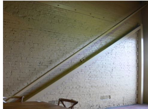
(b) wall strengthening using steel sections
