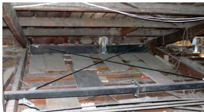
(e) roof diaphragm strengthening
