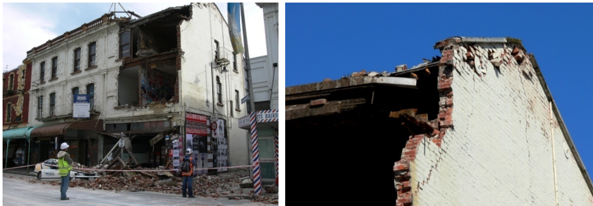
(a) 135-139 Manchester Street, out-of-plane facade collapse
