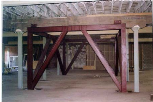
(b) Eccentrically braced core
