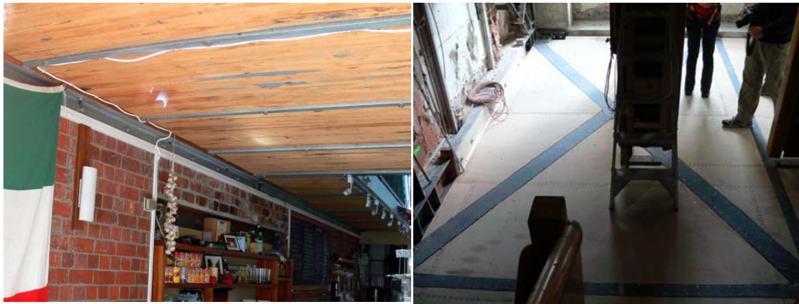
(a) Steel sections added to stiffen and secure the floor diaphragm (b) Steel strapping for floor stiffening
