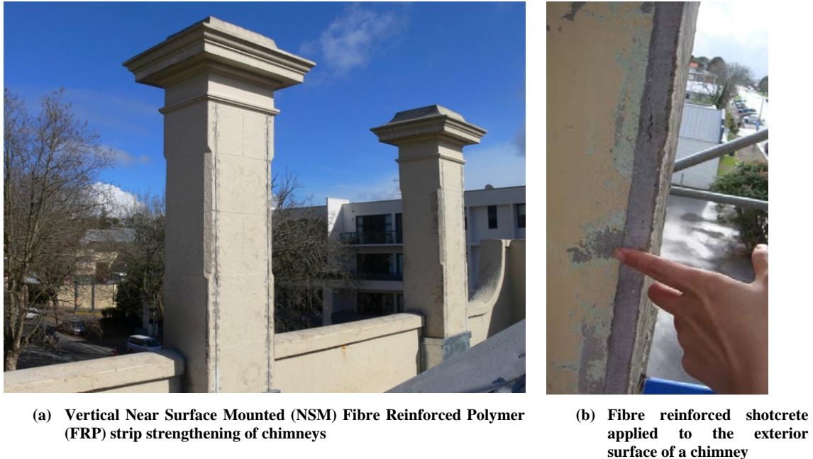
Figure 4.5 Examples of earthquake strengthened chimneys
