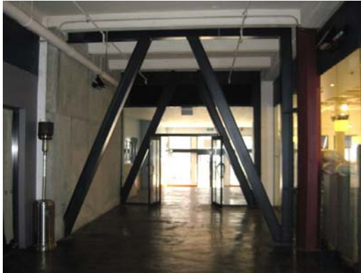
(a) Eccentric bracing in a walkway
