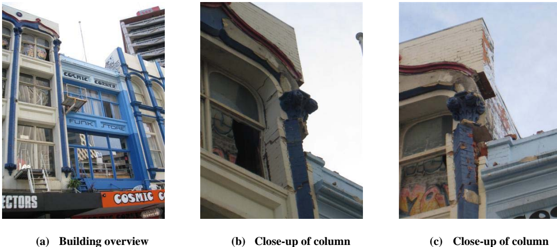
Figure 3.22 Example of building pounding damage
