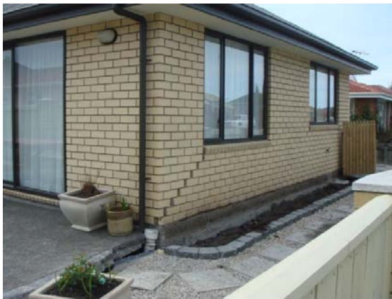
(c) Masonry veneer damage to recently built residence.
