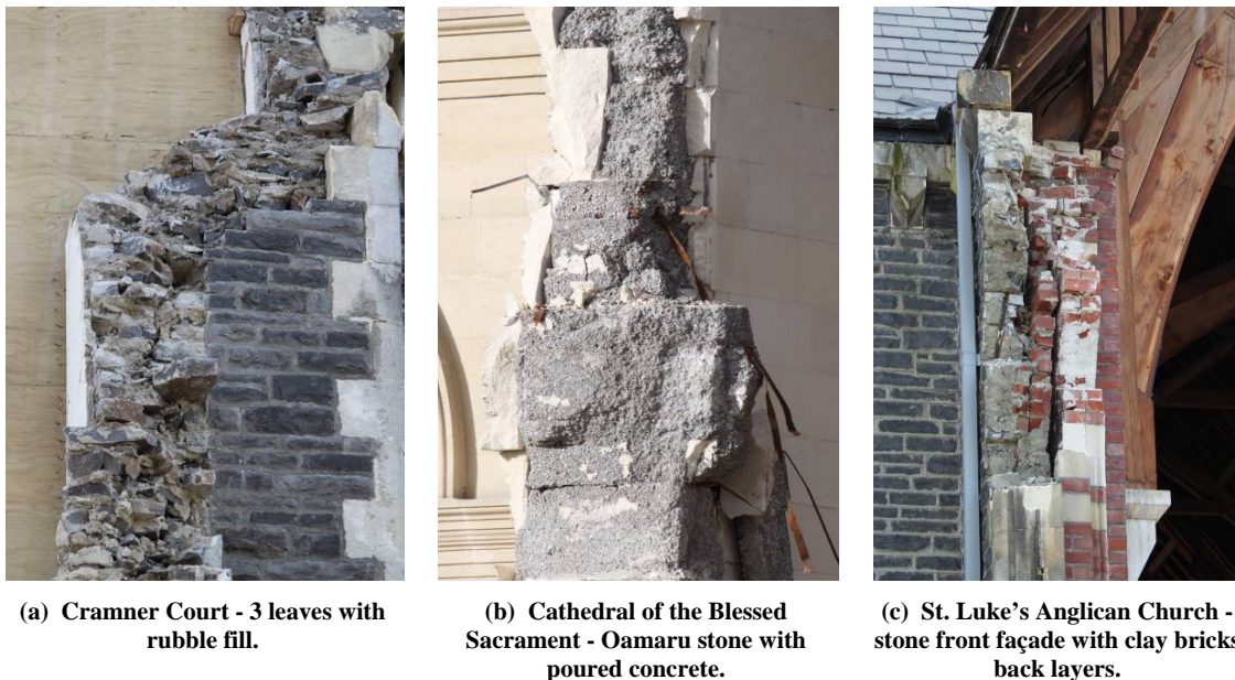
Figure 3.27 Representative examples of wall cross-sections for Christchurch stone masonry buildings
