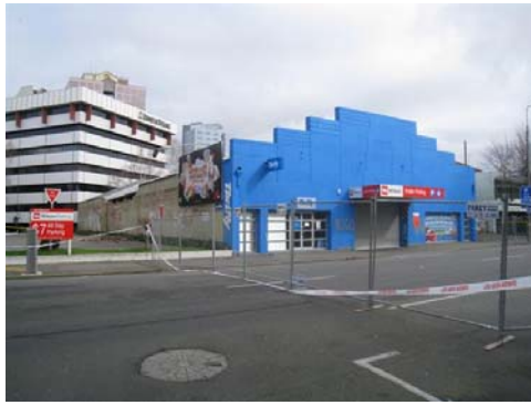
(a) Overview of building
