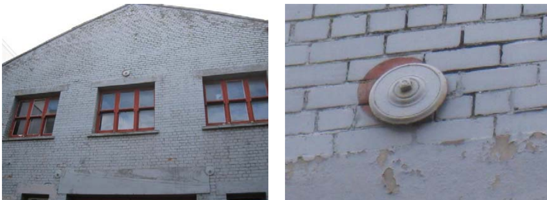
(a) Overview of wall anchors
