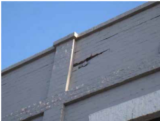
(c) Onset of anchorage failure
