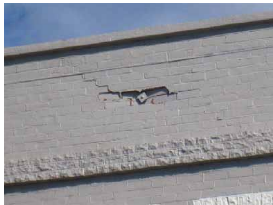
(b) Detail of partial anchorage failure
