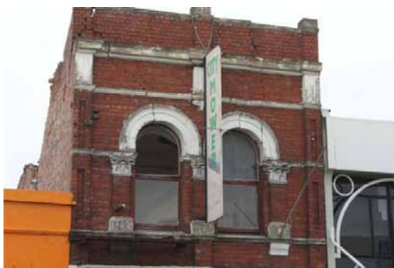
(a) Extensive vertical cracking above window openings
