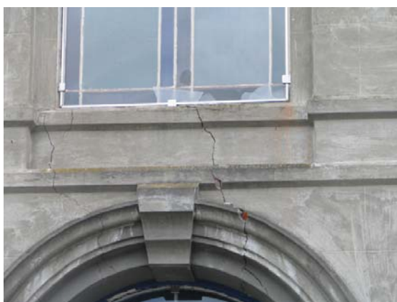
(c) Vertical crack through spandrel
