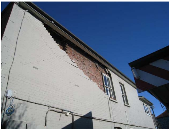
(c) Butterfly wall ties still intact
