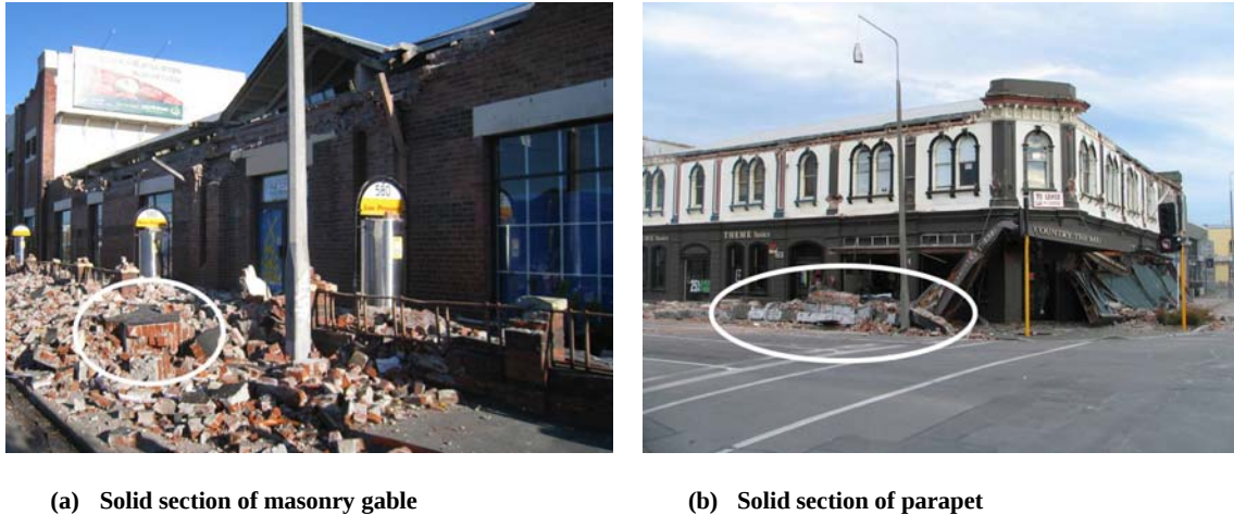
Figure 3.4 Large sections of masonry intact after fall from buildings
