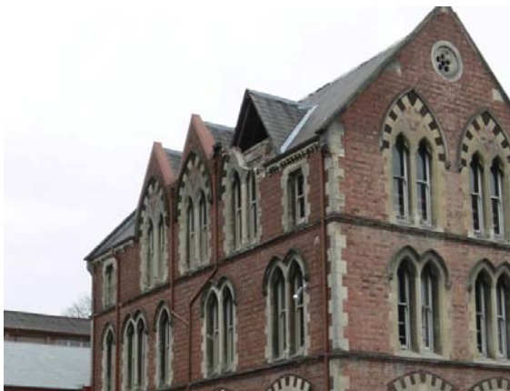
(c) Montreal-Armagh street corner
