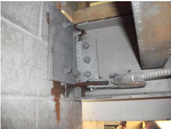
South East Corner Attachment – no damage
