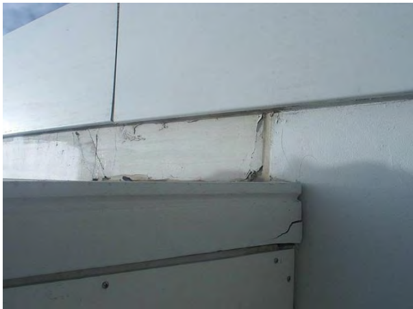
West balcony - west side
