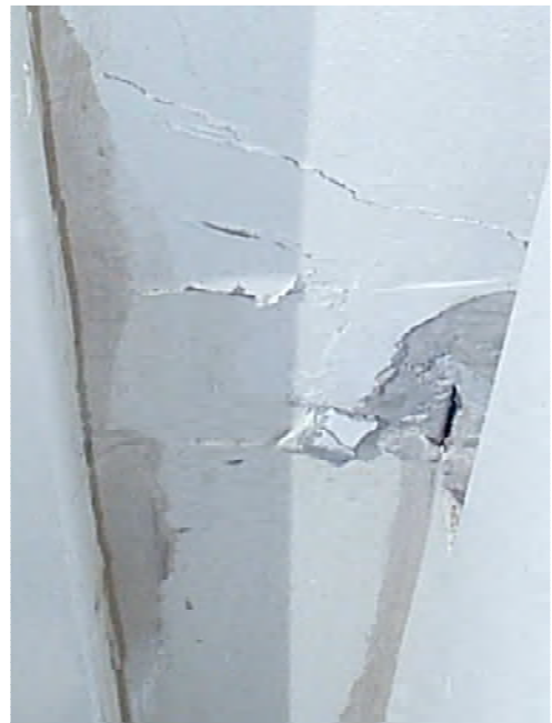
16 East Exterior Corner
