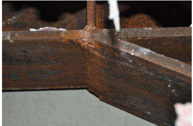
L6, Grid C2, brace weld
