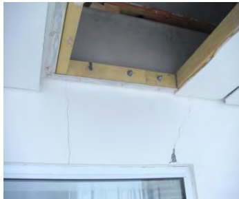
North Side East Level 11 Balcony
