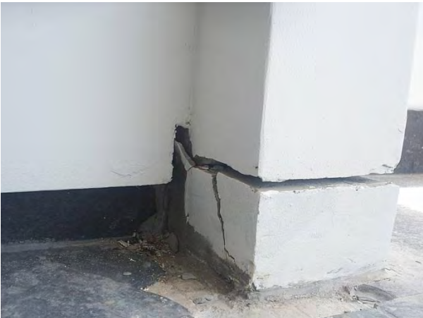
East balcony - west
