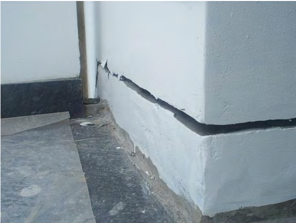
East balcony - east
