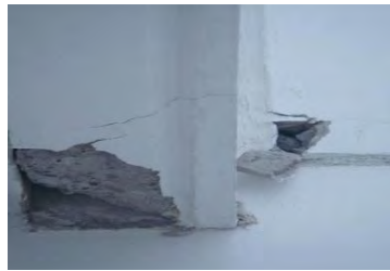
North Side Level 11 East underneath balcony
