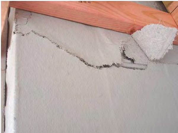
Southwest corner internal wall
