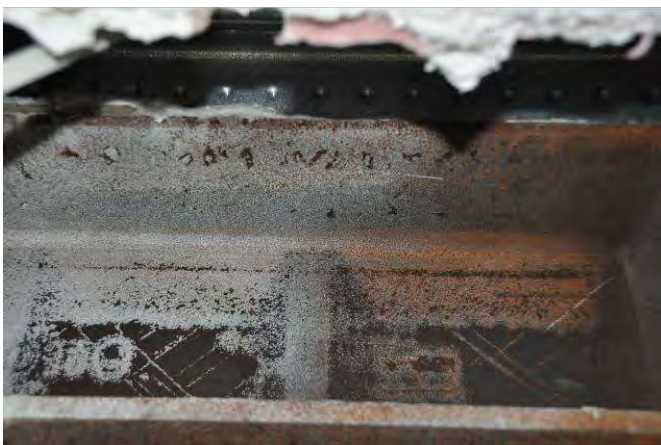
L7, Grid C2, Lueder's lines to active link
