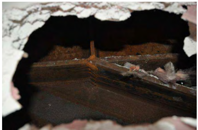
L6, Grid C2, brace weld
