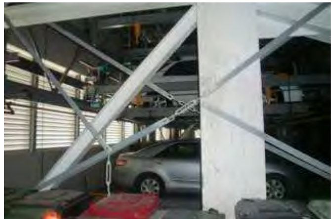
L2 Carstacker crossbraces "unhooked"
