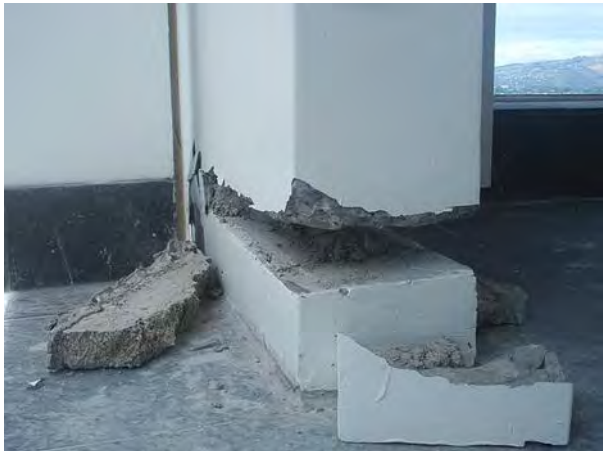
East balcony - east
