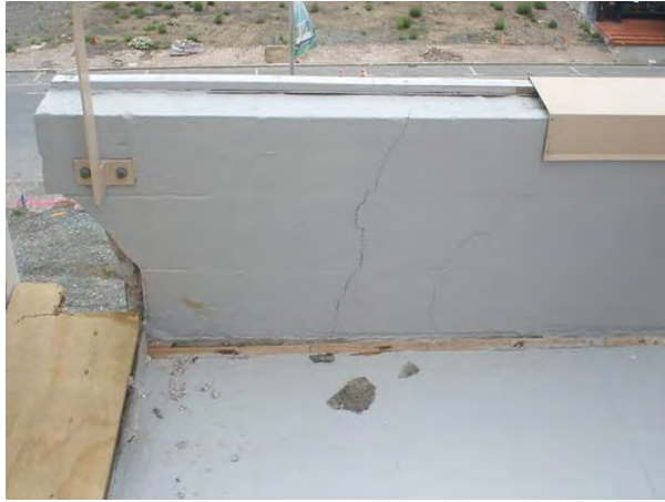
Southeast corner internal Parapet wall
