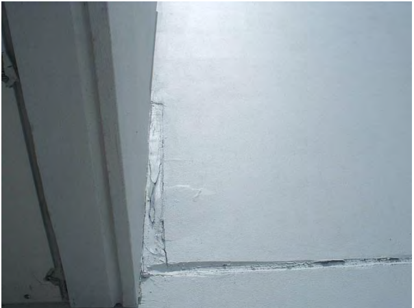
East balcony - west side
