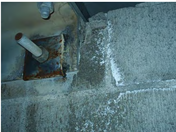
Mostly Fractured Concrete Block & Base Mount Bolt Mounts below Roof
