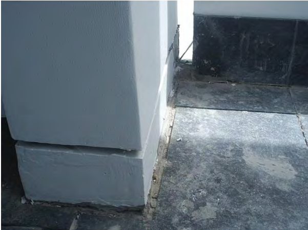
East balcony - west
