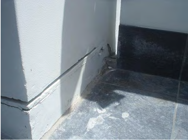
East balcony - west
