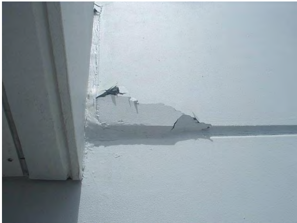
East balcony - east
