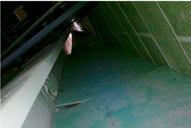
Flashings between masonry block and tower
