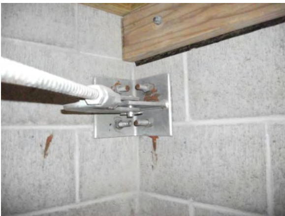
South West Attachment – no damage
