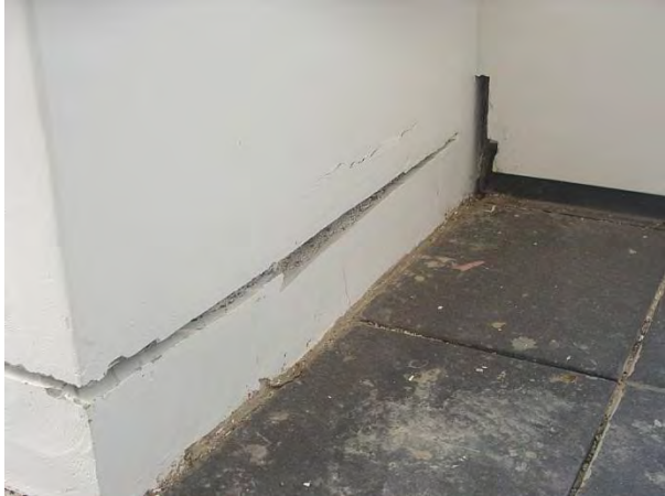
East balcony - east
