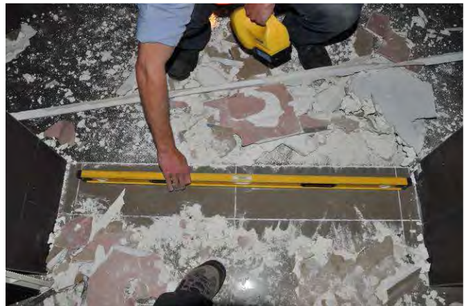
L7 floor at Grid C1/26, essentially level
