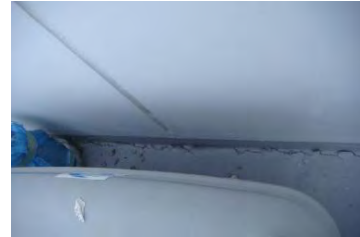
North Side Level 11 Deck
