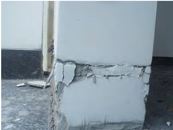
East balcony - west
