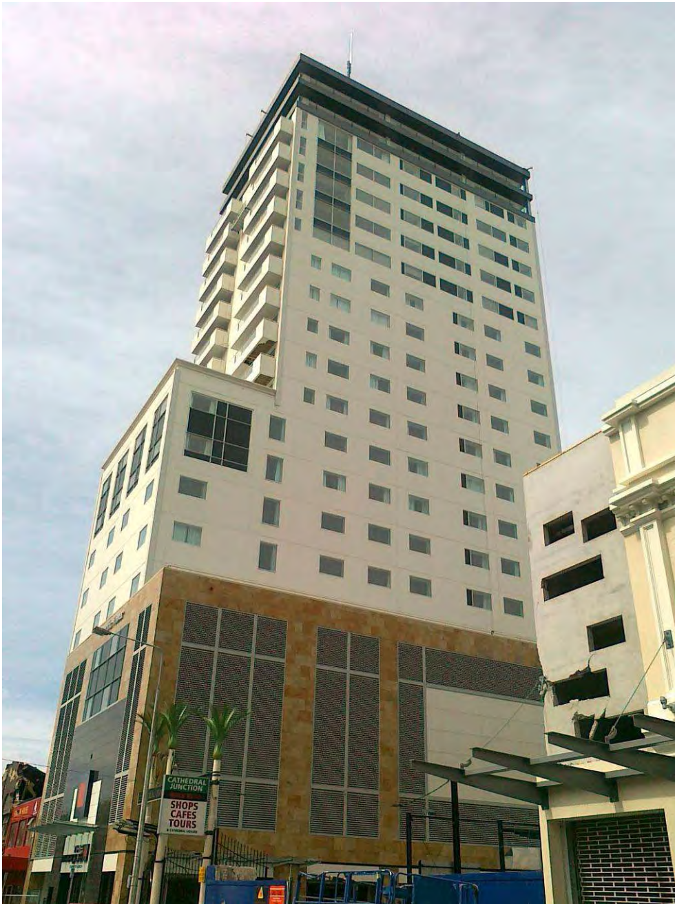
Pacific Tower 2 March 2011 (some damage to north balcony soffits visible).
