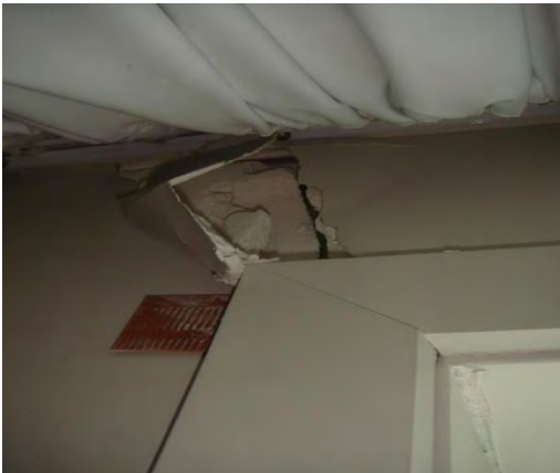
Nth - Sth Battering Ram I Beam Effect Sth Room #921
