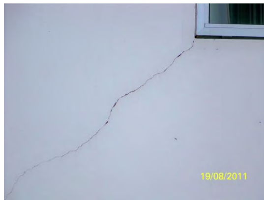
Level 10 Left Side of Window, Rt Panel
