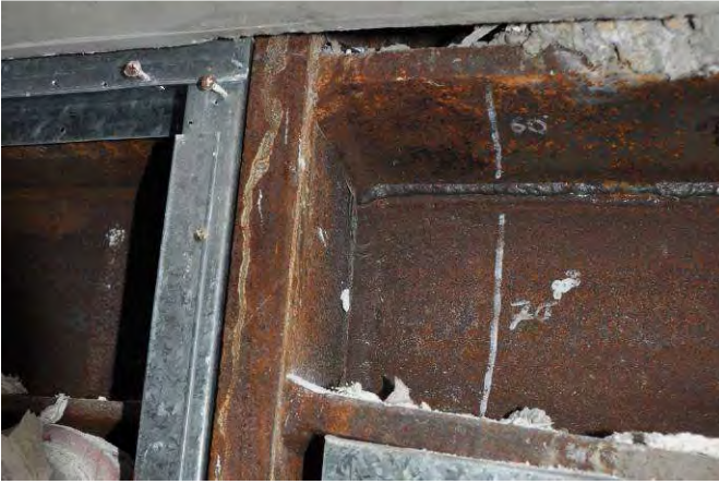
L11, Grid D4, column joint
