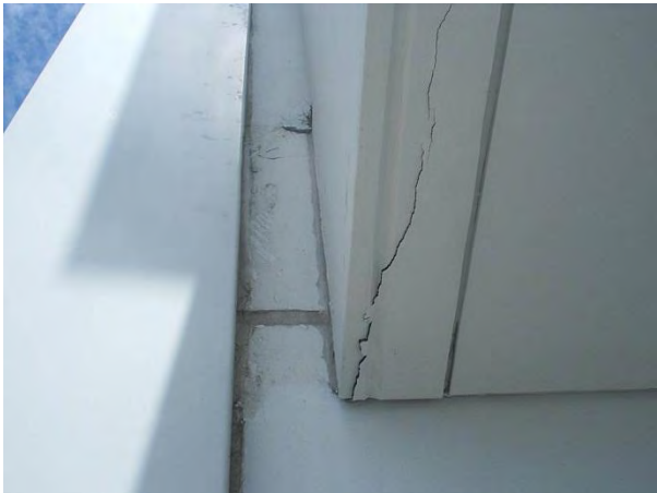
East balcony - east
