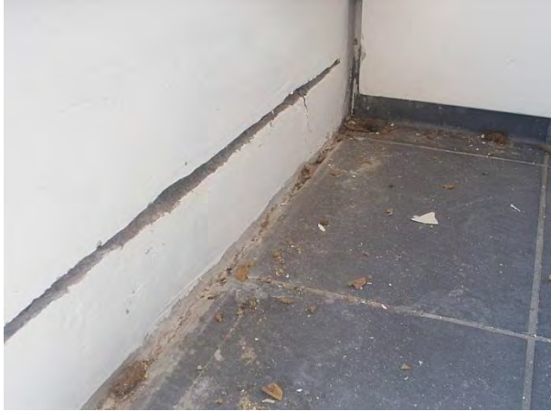
East balcony - east
