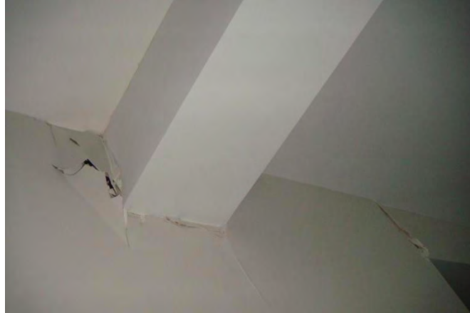
Sth Room # 801 - Nth - Sth Movement Battering Ram Effect
