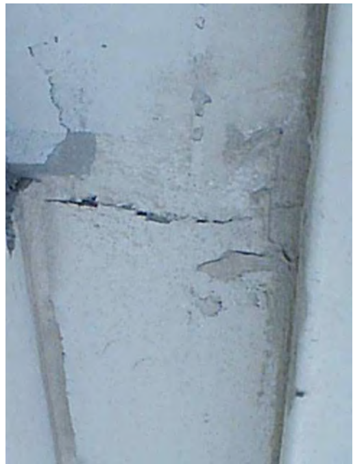
16 West Exterior Corner
