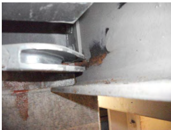
North East Corner Attachment – no damage
