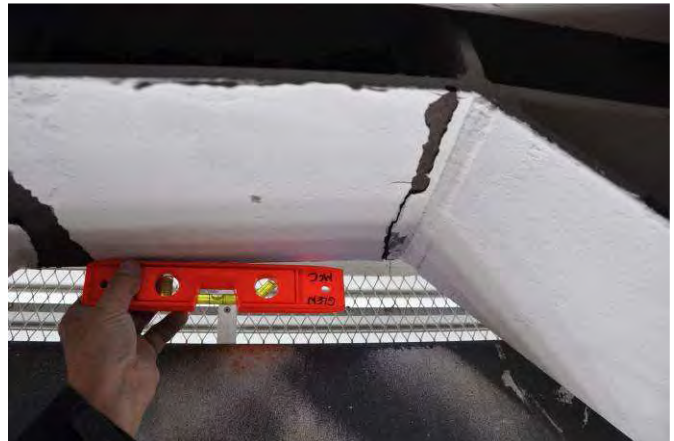
L2, Grid E½1, active link, permanent offset
