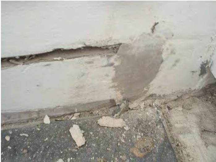
16 East Interior Corner
