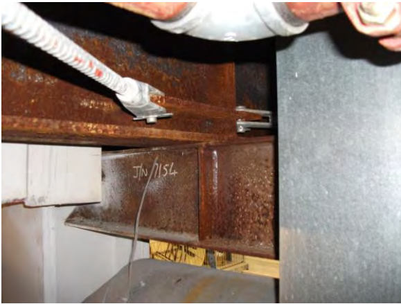
South West Corner Attachment – no damage
