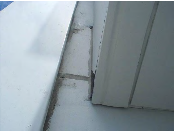
East balcony - east
