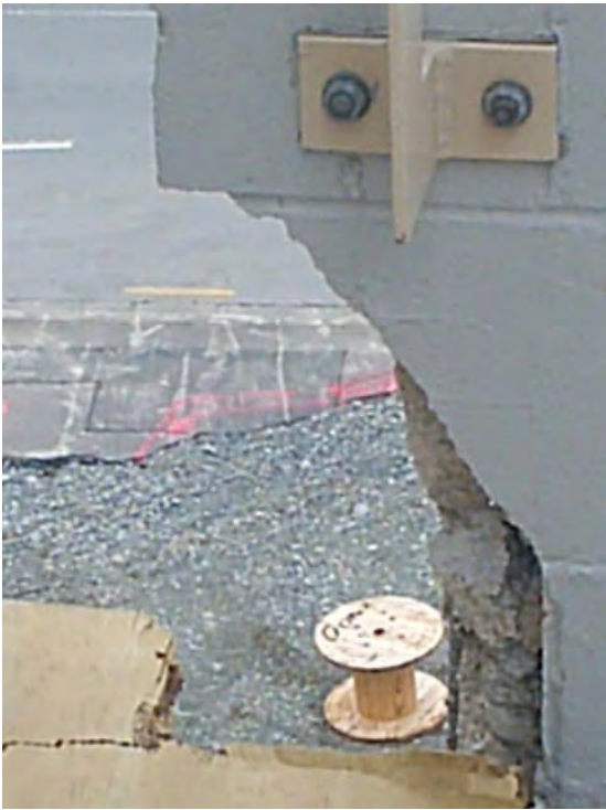
Southeast corner internal Parapet wall
