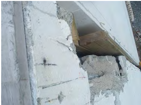
Southeast corner external wall
