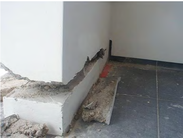
East balcony - east
