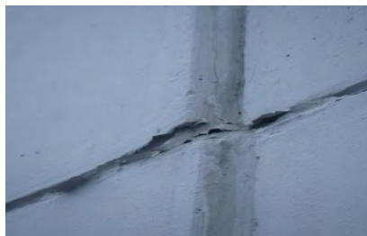
Level 12, Nth Side, Between Balconies
