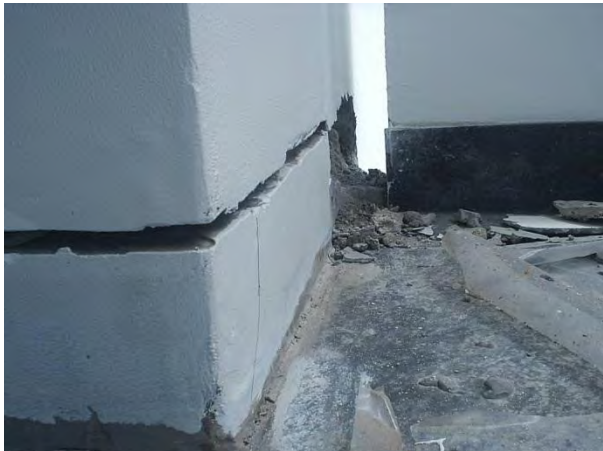
East balcony - west
