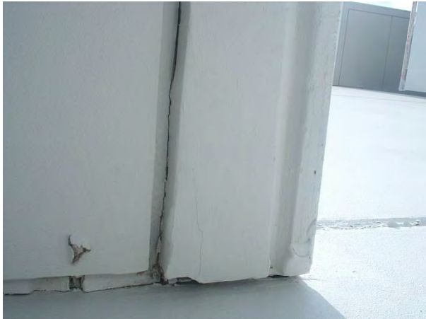
East balcony - west
