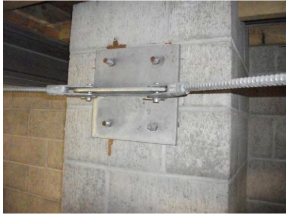
Central South Side Plate Attachment – no damage
