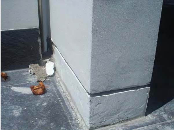
East balcony - east
