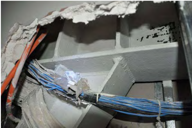
L6, Grid D4(east), brace weld
