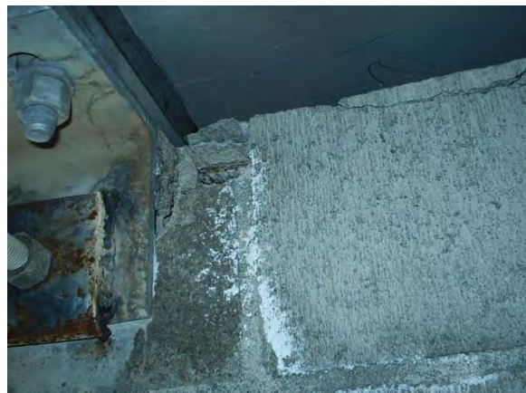
Mostly Fractured Concrete Block & Base Mount Bolt Mounts below Roof
