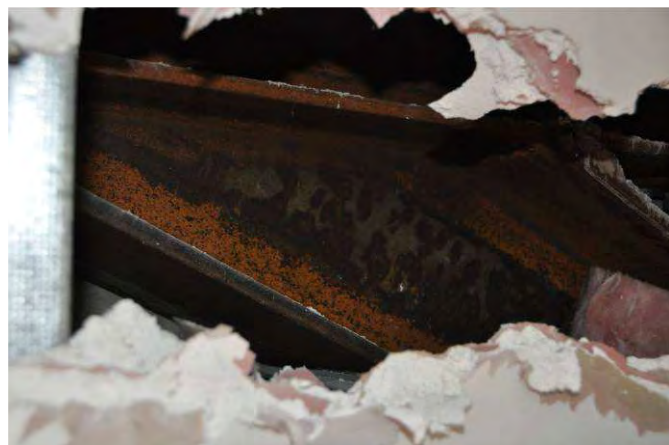
L7, Grid C2, brace connection
