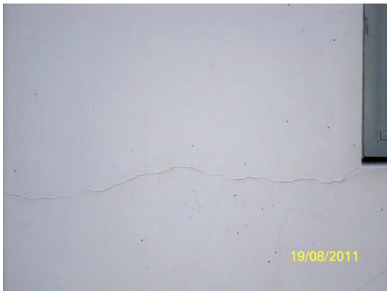
Level 8 Right Panel
