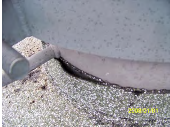
Top Base Roof Ring Water Seal Broken
