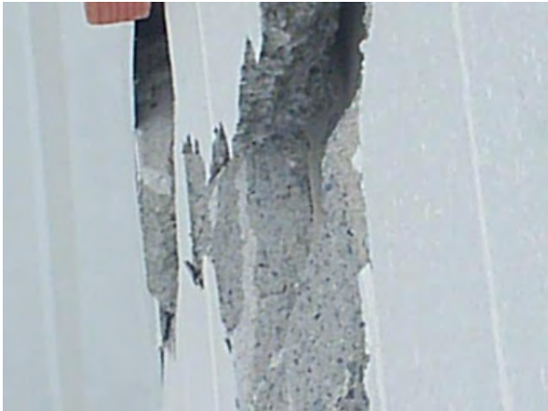
Southwest corner external Parapet wall
