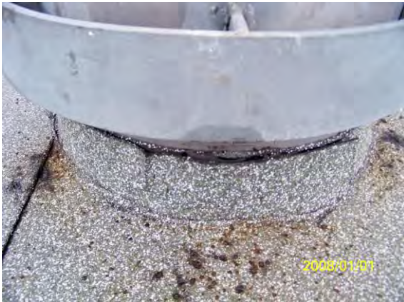
Top Base Roof Ring Water Seal Broken
