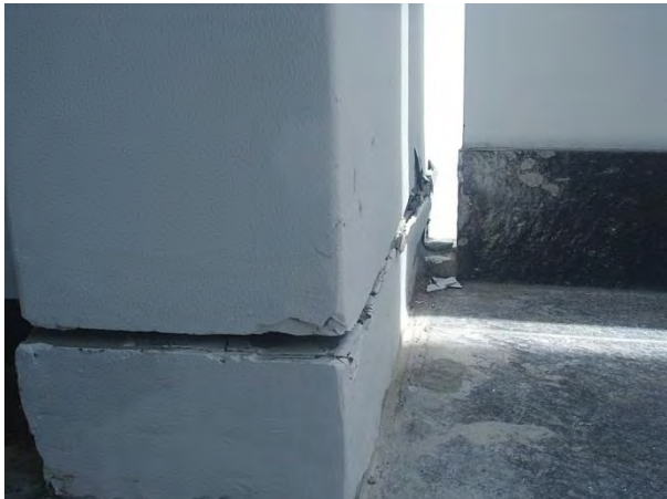
East balcony - west
