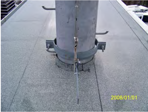
Top Base Roof Ring Water Seal Broken
