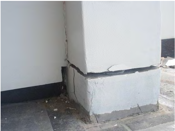
East balcony - west
