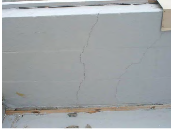
Southeast corner internal Parapet wall
