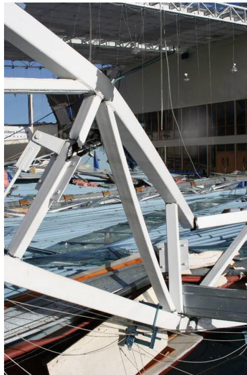
Figure 28 - Truss T4 prior to being moved on 25 September 2010 (clockwise from top); (a) View from south wall; (b) Top chord splice without packer plate failure and reduced wall thickness bottom chord failure zones at quarter point. Diagonal rod bracing cleat has pulled out of vertical strut on eastern side; (c) View from northern end of Truss 4 showing westward offset from mid-span
