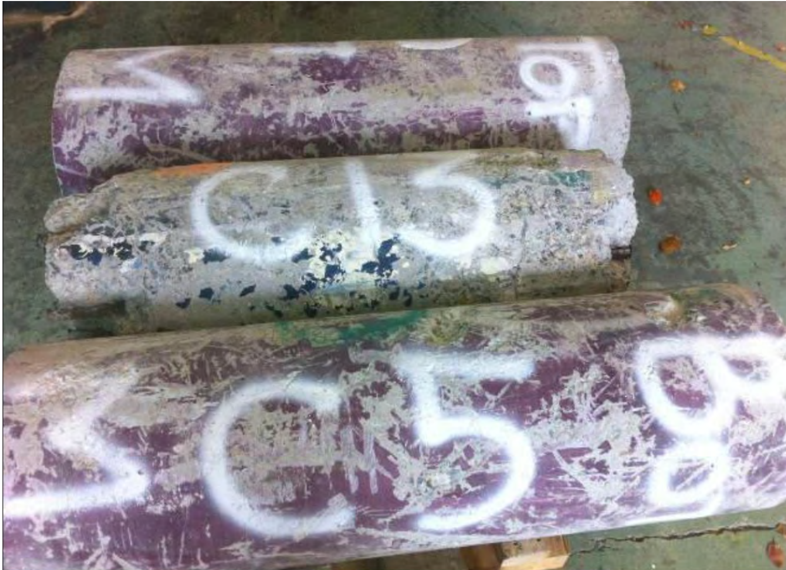
Fig. 2.4. The three column portions retrieved from the CTV Building used in the full-scale testing conducted at the University of Canterbury
