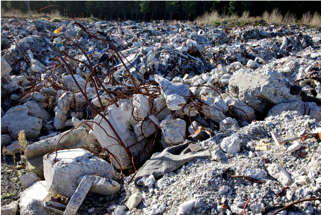
Figure 1 Remains of CTV Building at Burwood
