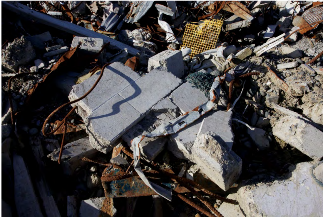
Figure 3 Remnant of 140 mm block wall
