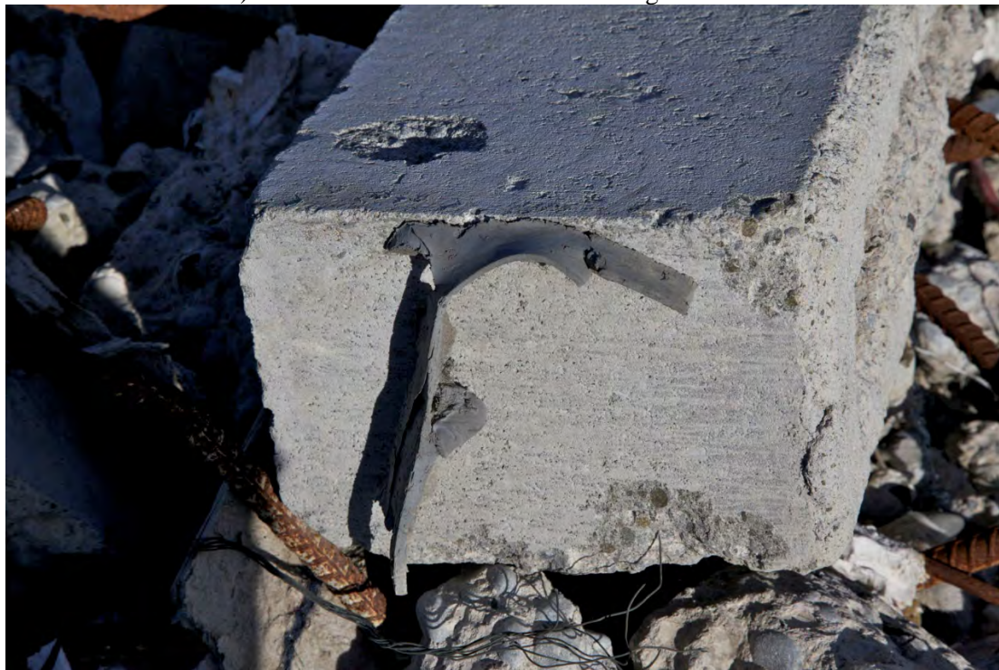
b) Remnant of sealant on reinforced core filled blocks
