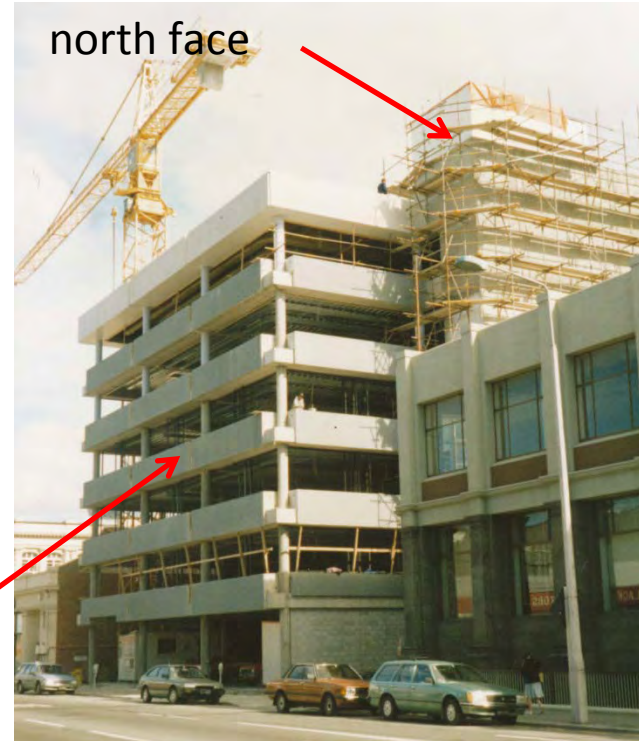
Pre-cast concrete Spandrel panels between columns on edge beams
