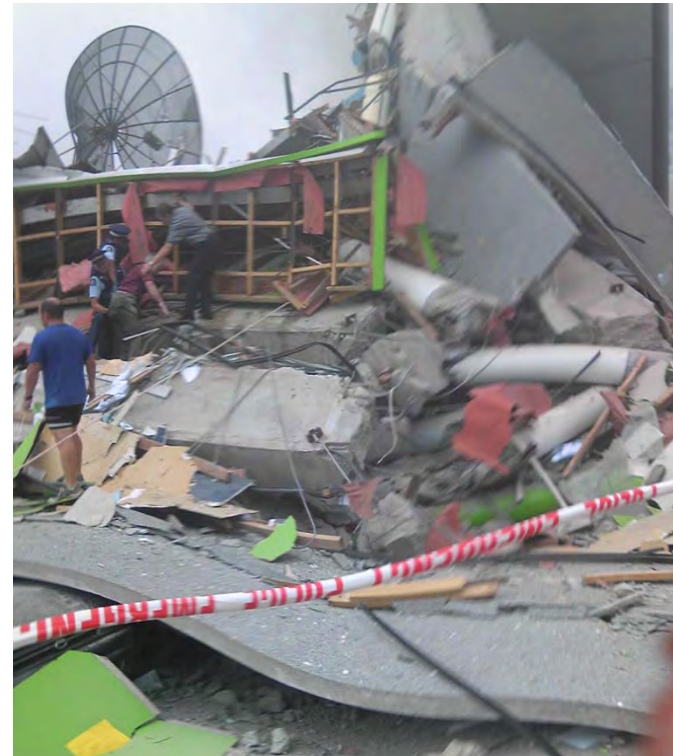
View from east at Line 4 North Core immediately after the collapse at 1:00 pm
