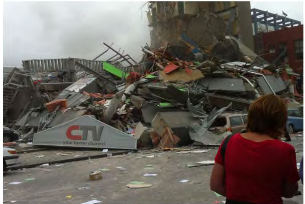
View from southeast Immediately after the collapse
