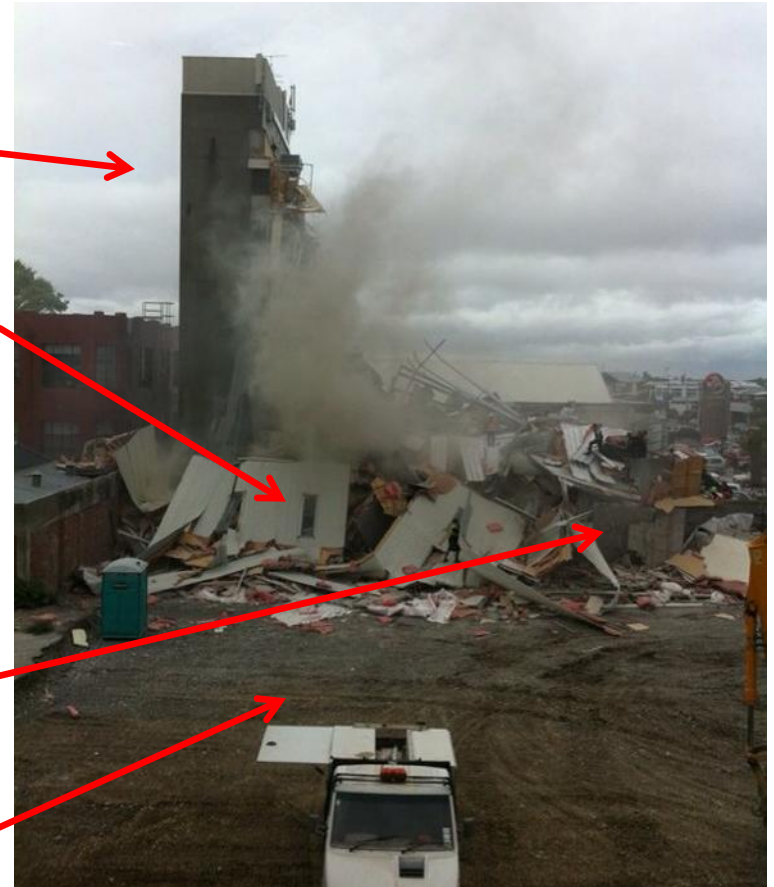
View from Les Mills from west Immediately after the collapse
