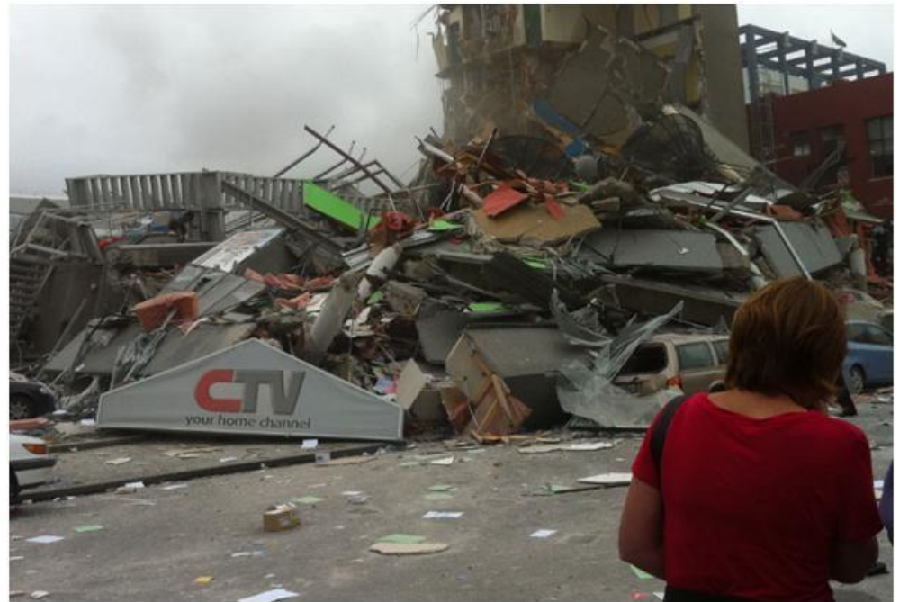
View from southeast Immediately after the collapse
