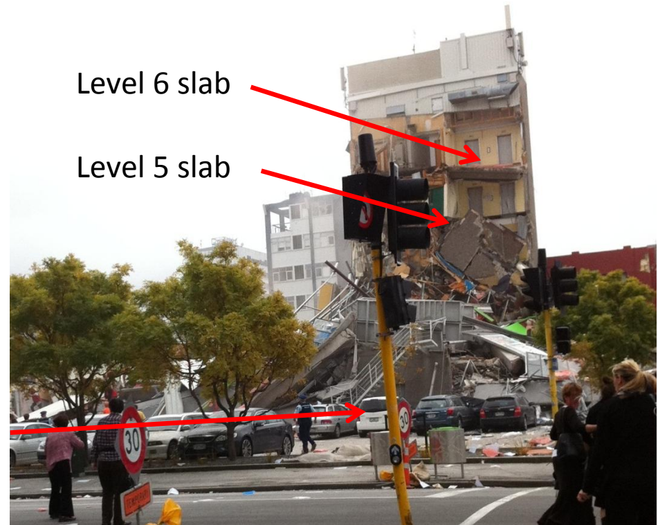
View from Cashel Street from south Immediately after the collapse
