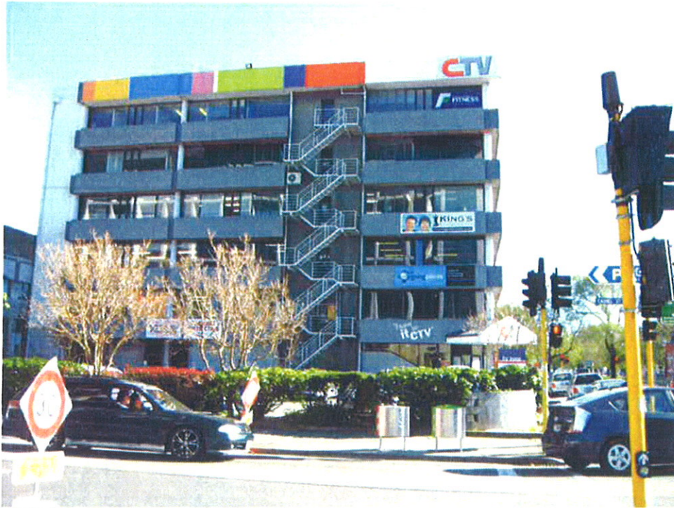
Photo 1 South Elevation of Building
