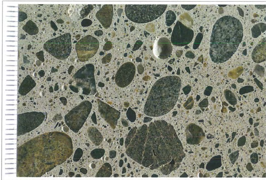
Figure F7. Photograph of the polished surface showing coarse aggregate; scale in millimeters.
