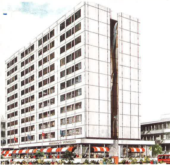
1. Durham Towers Hotel, cnr Durham and Gilmore Streets, Christchurch.
