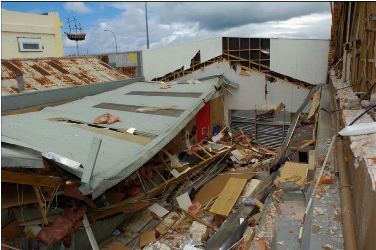
Figure 4: Damage to single-storey building from failure of upper level wall and parapet from neighbouring building at right (Photo from Gisborne Herald)
