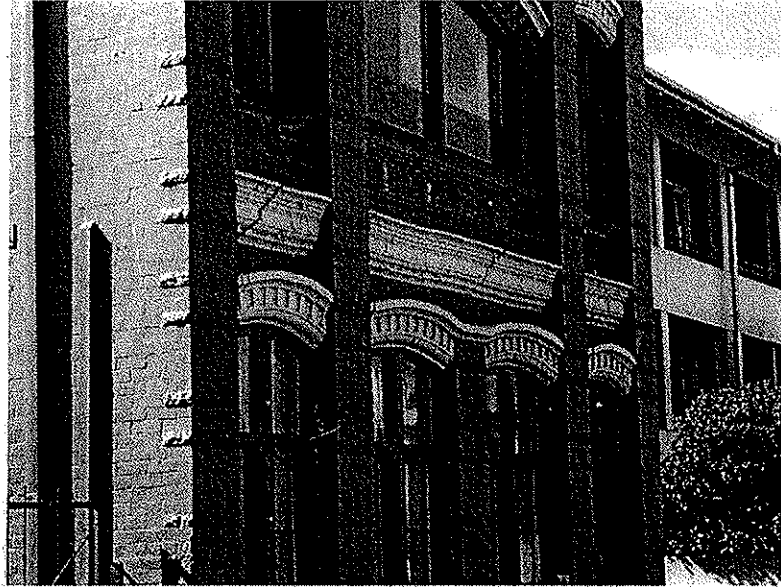
Figure 9: West Facade 15 Feb - note out-of-plane offset of near lintel
