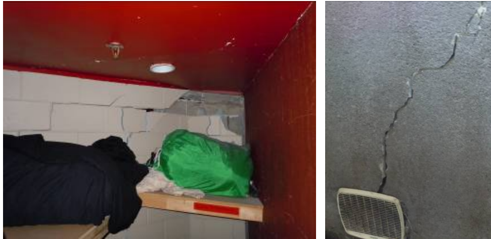
Figure 9: Typical Block Wall Damage (left) and Concrete Shear Wall Cracking (right) [1]
