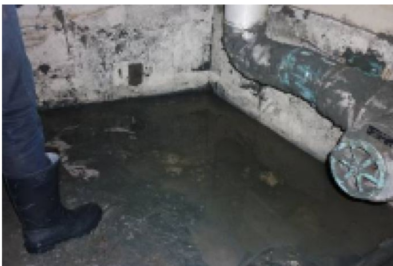
Figure 15: Evidence of Liquefaction in Basement [1]
