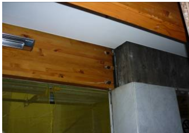
Figure 13: Glue-Laminated Beam Connection Tear-Out [1]
