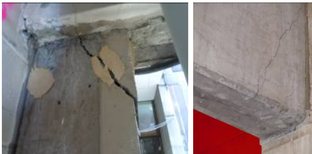
Figure 10: Column Cracking (left) and Beam Cracking (right) [1]
