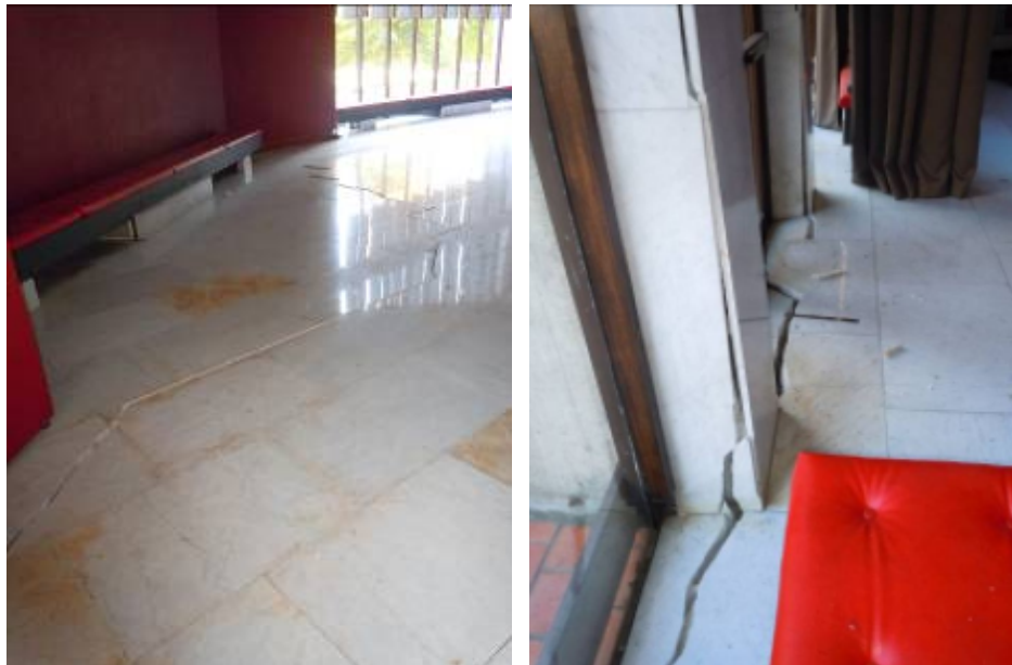
Figure 11: Slab-on-grade Damage [1]
