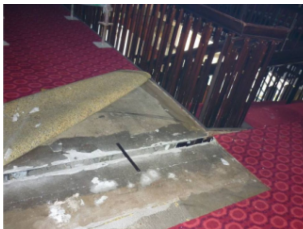
Figure 8: Building Joint Damage [1]
