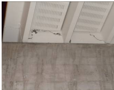
Figure 14: Double-Tee Cracking [1]
