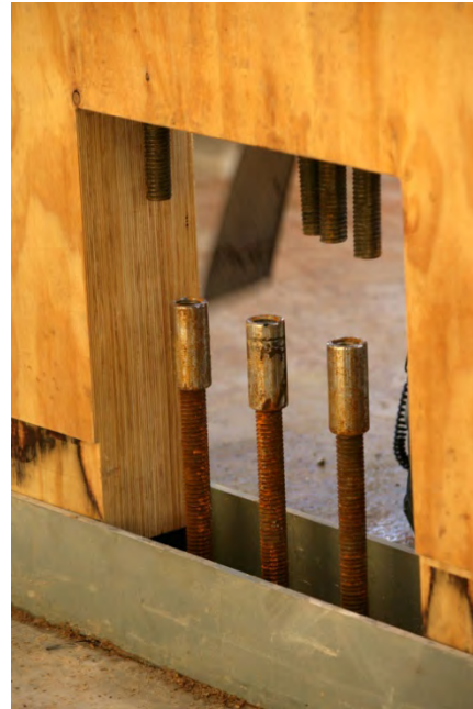
Post tensioned steel
