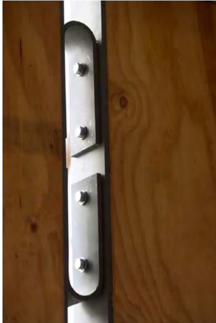
Seismic Energy Dissipators
