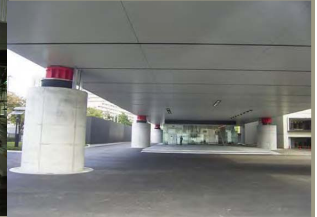
Lead-rubber bearing
