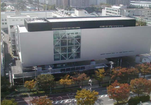
Six columns can uphold the entire building
