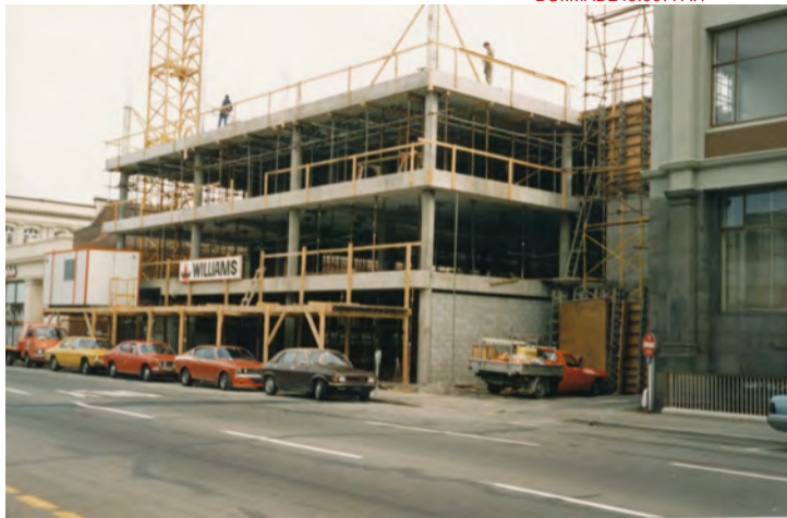
Construction of CTV building 1987
