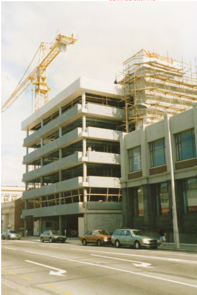
Construction of CTV building 1987
