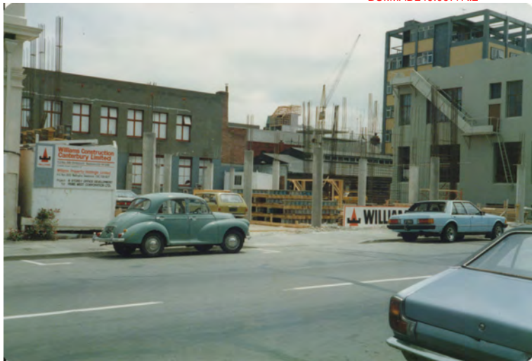
Construction of CTV building 1987
