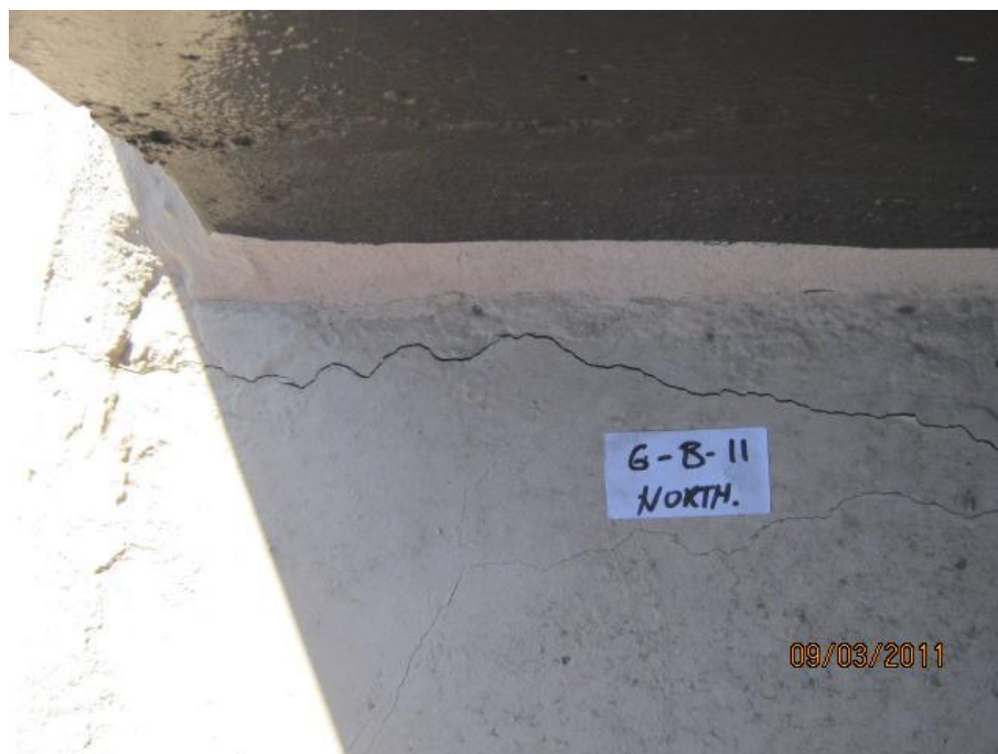
Figure 14: Example of beam cracking (Grid B3 Level 6, from [11])
