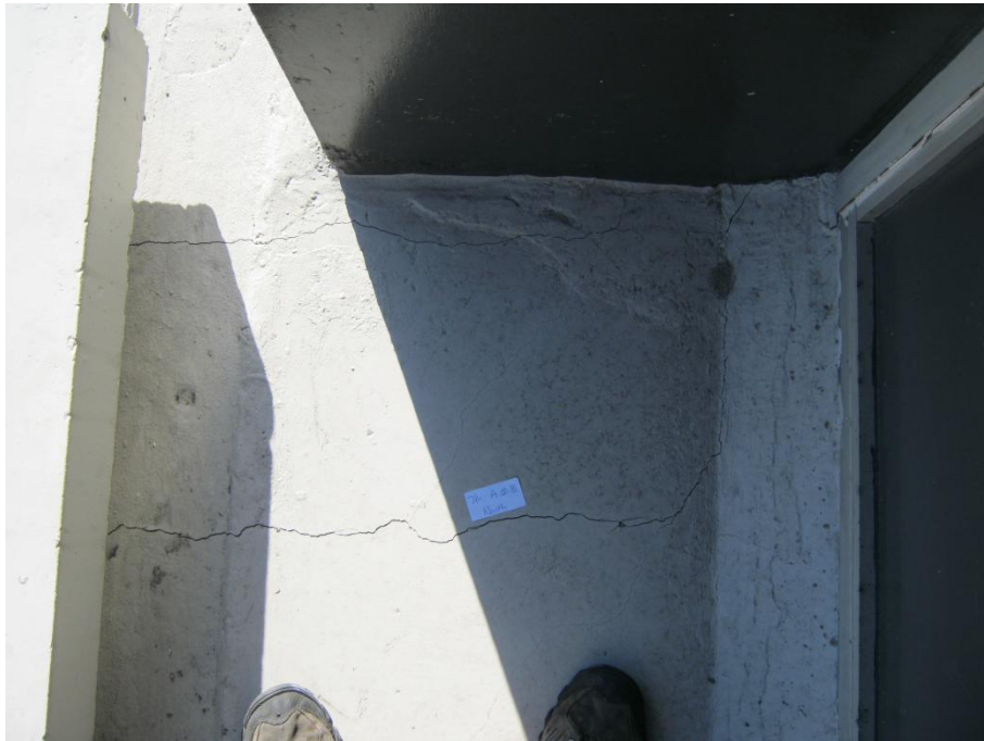
Figure 15: Example of beam cracking (Grid B2 Level 7, from [11])
