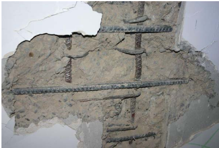
Buckling of vertical reinforcement level 2
