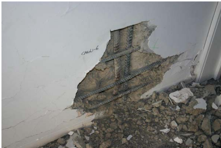
Buckling of vertical reinforcement level 1
