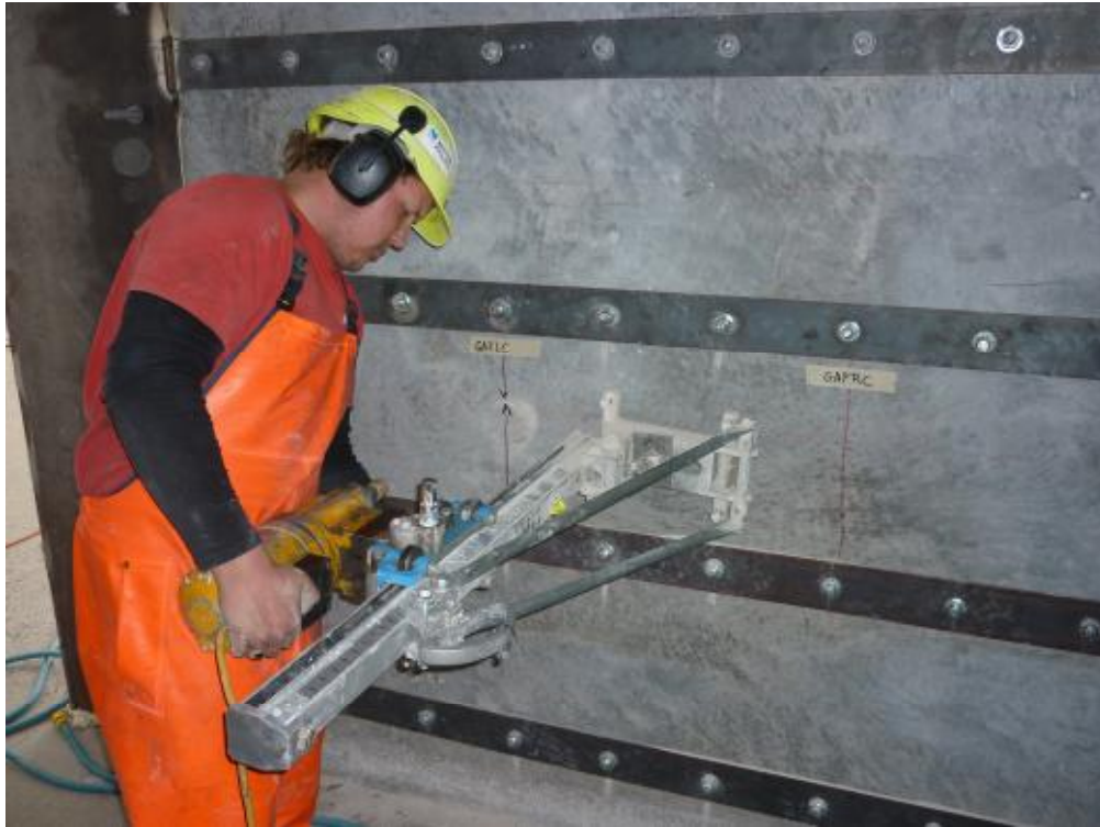
Figure 1 Drilling concrete core from Gallery Apartments
