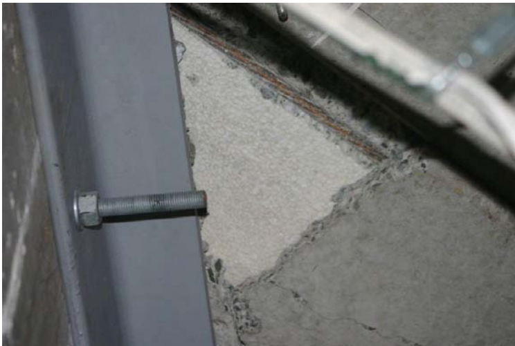
Spalling of Dycore concrete has exposed the pre-stressing strand
