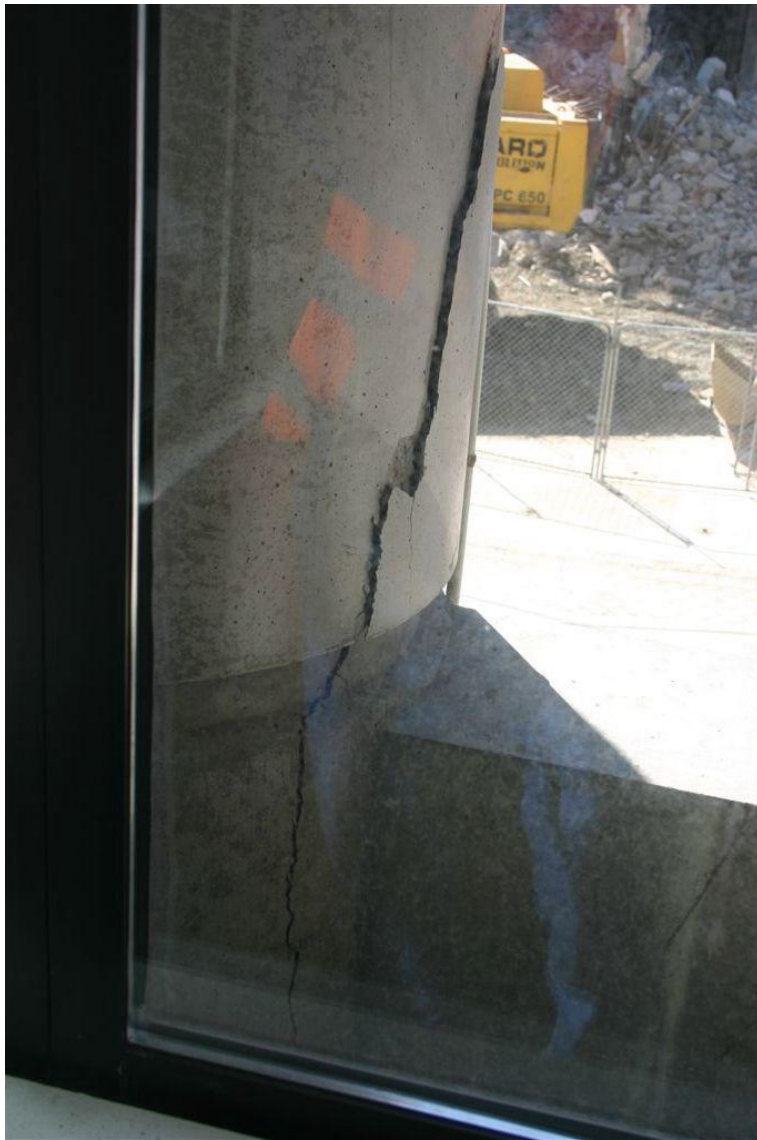
Spalling of circular external column
