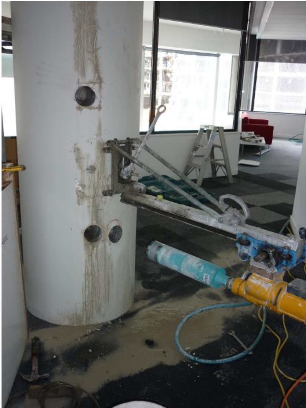
Figure 5 Core Drilling in concrete column
