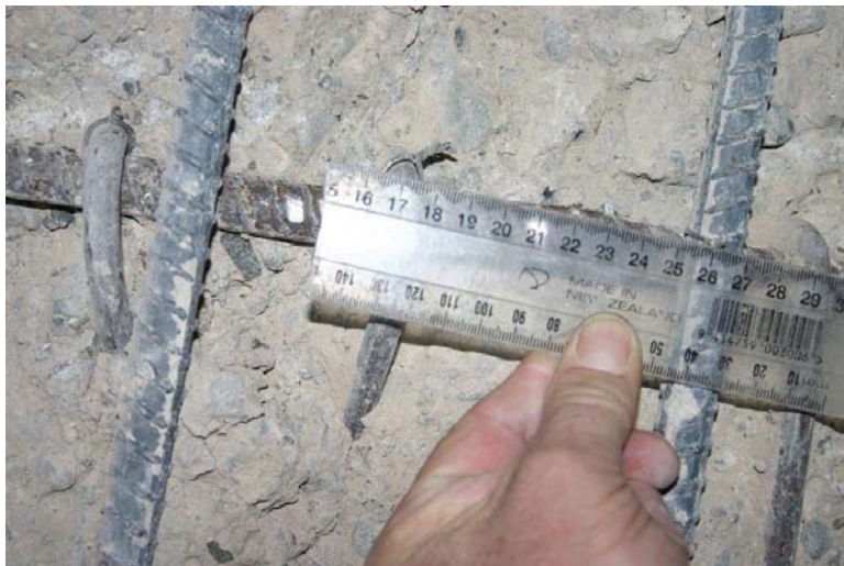
Variation in spacing of restraint at location where reinforcement has buckled
