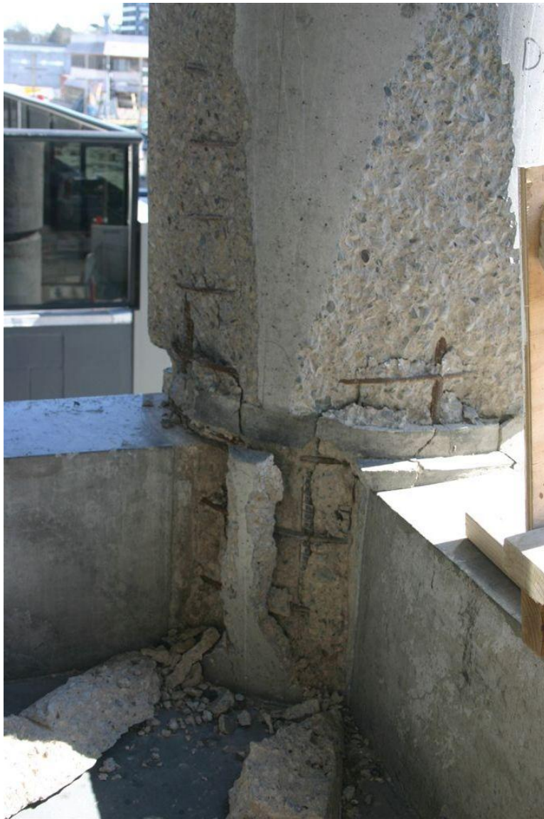
Spalling of circular external column
