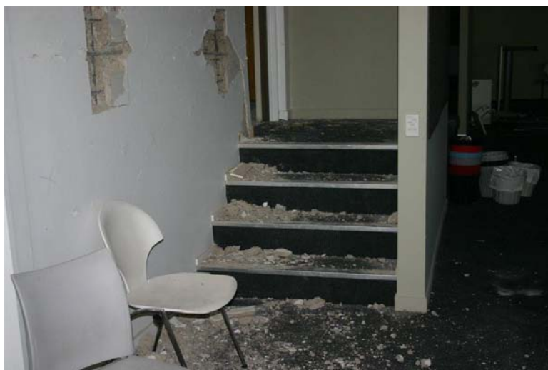
Spalling of shear wall level 2
