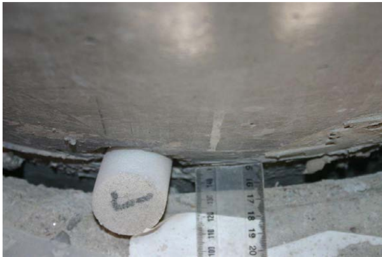
Tearing between pre-cast truss and floor
