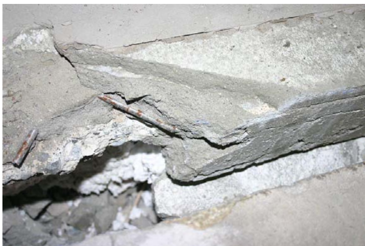
Damage to seismic joint
