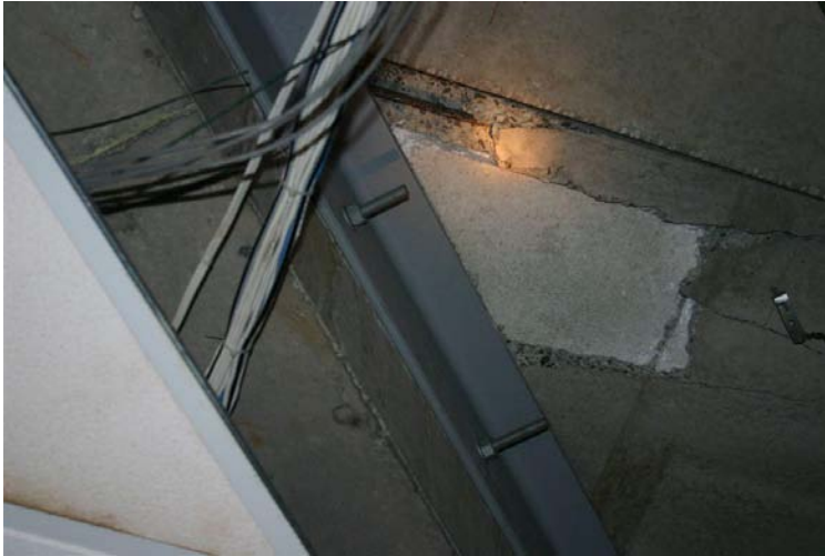
Retrofitted steel angles for seating of Dycore floor units
