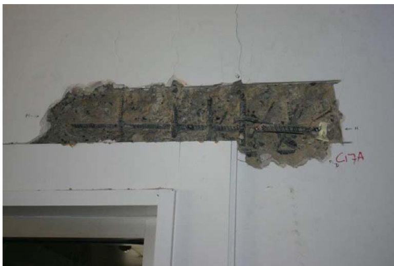
Buckling of reinforcement at corner of shear wall coupling beam
