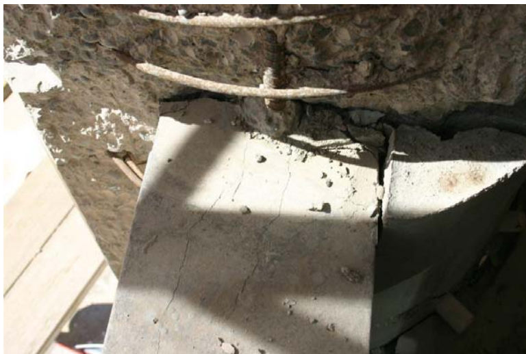
Spalling of circular external column at junction with pre-cast truss
