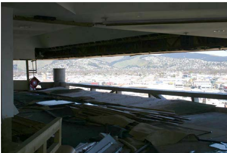
View of roof structure cantilevering out from the shear core
