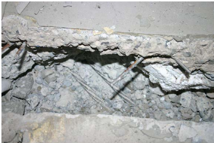
Damage to seismic joint
