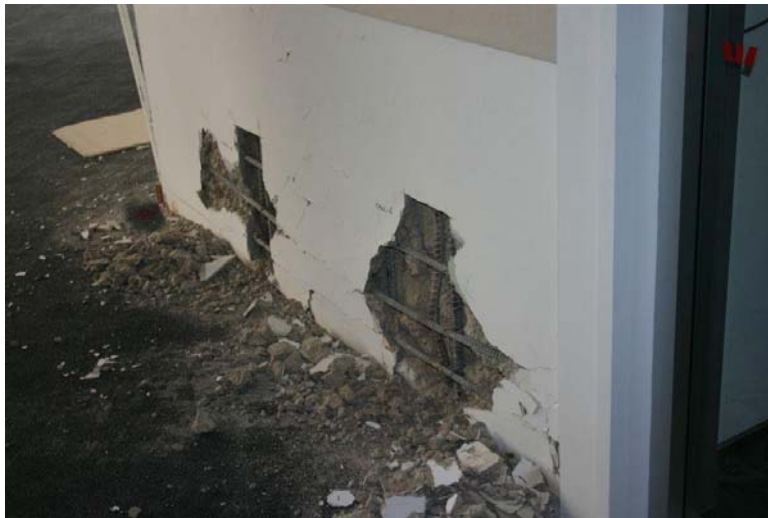
Spalling of shear wall level 1
