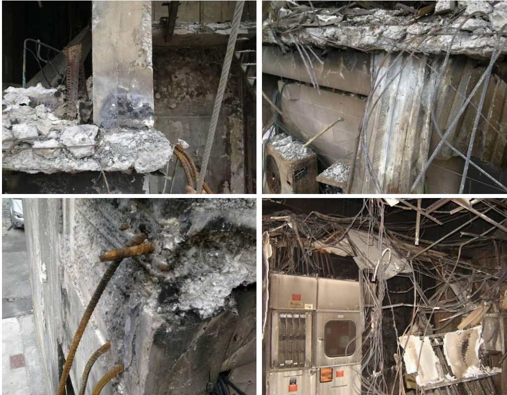
Figure 31 - Line 4 North Core Walls Level 2 slab remnants (clockwise from top left) (a) Slab edge broken back during de-construction adjacent to stairwell wall; (b) Broken back slab with H12 saddle bars exposed. Masonry wall with separation along top course; (c) Switch room under Level 2 slab; (d) Connection of shell beam to wall with two fractured H24 top bars and one de-bonded top bars. Bottom bars from shell beam have been embedded in wall as specified (DENG B23 Dwg S18 (Figure 67), Detail 5 S19 (Figure 71)). Some diagonal beam-wall joint zone shear cracking can be seen in the wall end..
