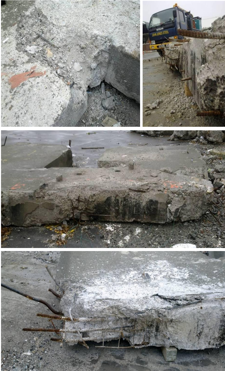
Figure 22 - Line I South Wall Level 5 to Level 6 (Item E5) (clockwise from top left) (a) Crumbly concrete at door edge of west pier able to be dislodged by boot; (b) Smooth and charred construction joint on top west surface looking east; (c) Charred construction joint above west pier. Door sill on left; (d); Top east corner with fractured top 3-H24 bars. Floor 664 mesh exposed.
