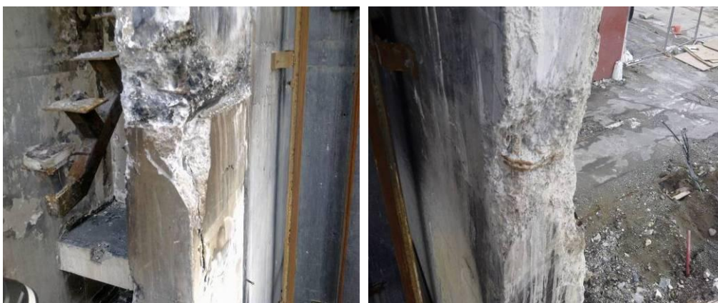
Figure 34 - Level 2 Lift Well Wing Walls Grid D and D/E (left to right) (a) 20 mm hole in end where a reinforcing bar has pulled out of wall. 200 mm thick construction joints in wall at slab level; (b) No reinforcing steel attachment into the east wing wall at Level 2
