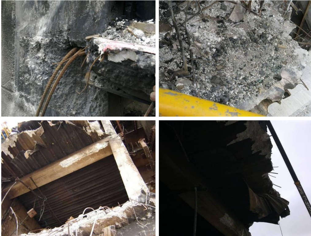
Figure 30 - Line 4 North Core Walls Level 3 slab remnants (clockwise from top left) (a) Connection of shell beam to wall with two fractured H24 top bars and two de-bonded top bars. No bottom bars from shell beam embedded in wall but imprints from bars evident (DENG B23 Dwg S18 (Figure 67), Detail 5 S19 (Figure 71)), corresponding to the bent back bottom steel in shell beam Item E23 (Figure 8); (b) Ash on slab;. Cored holes at fractured edge; (c) Torn profiled metal deck sheeting de-bonded from slab but still fixed in at pre-cast beam support (DENG B24 Dwg S18 (Figure 67)); (d) Profiled metal deck and slab from below supported on beam B24.
