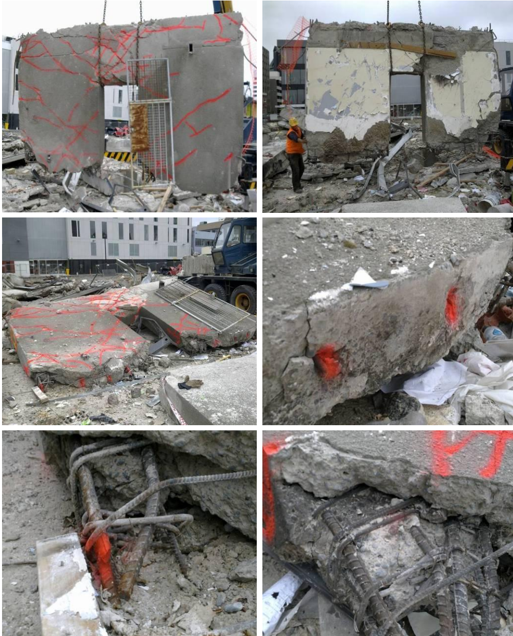
Figure 16 - Line 1 South Wall Level 2 to Level 3 (Item E2) (clockwise from top left) (a) Outside face with fire escape door attached. Cracks marked by red paint; (b) Inside face of wall; (c) East pier construction joint with necked and fractured bars indicated by red paint; (d) Escape door edge of east pier showing thick cover concrete to reinforcing; (e) Outer edge of west pier showing necked and fractured bar indicated by red paint others were cut; (f) Outer face of wall with cracks and fractured bars marked.
