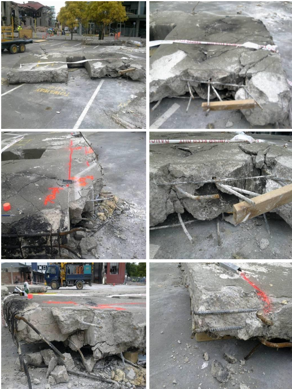
Figure 20 - Line I South Wall Level 4 to Level 5 (Item E4) (clockwise from top left) (a) Outer face with east pier on right with severe shear damage, and timber formwork remnant; (b) and (c) Charring on fractured concrete surfaces prior to deconstruction; (d) Top west corner showing saw-cut on top edge from deconstruction; (e) Top east corner showing smooth construction joint at interface with pre-cast beam B15 (DENG Dwg S18 (Figure 67)) and fire charring to spalled eastern edge; (f) View from east to west of top east corner construction joint notch.
