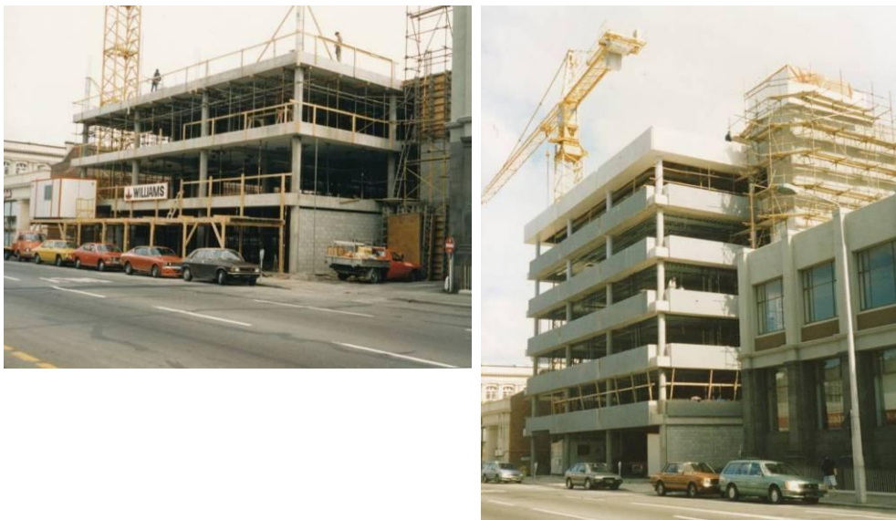
Figure 45 - CTV Building under construction (left to right) (a) May 1987 with floors cast up to Level 4; (b) October 1987 with roof on and pre-cast spandrel panels attached; Columns C21 to C23 had not been built at that time in the northeast corner closest to camera.
