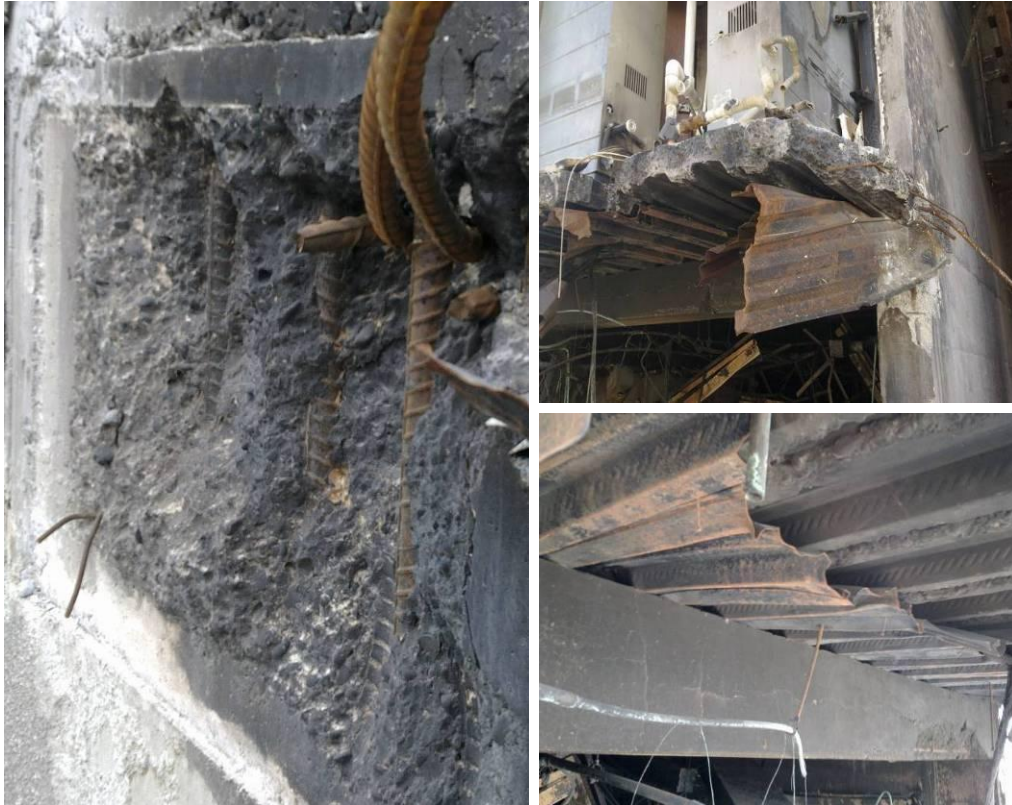
Figure 29 - Line 4 North Core Walls Level 4 slab remnants (top to bottom) (a) Connection of shell beam to wall with two fractured H24 top bars and two de-bonded top bars. No bottom bars from shell beam embedded in wall but imprints from bars evident (DENG B23 Dwg S18 (Figure 67), Detail 5 S19 (Figure 71)), corresponding to the bent back bottom steel in shell beam Item E23 (Figure 8); (b) Fractured vertical face of slab at stairwell wall, with fractured slab support beam (DENG B25 Dwg S18 (Figure 67)) top bar and charred fracture surface; (c) Torn profiled metal deck sheeting de-bonded from slab but still fixed in at pre-cast beam support.
