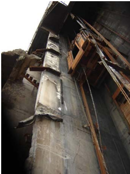
Figure 33 - Drag Bar connections at Levels 6, 5 and 4 on lift well west wing wall on Grid D. No Drag Bar at Level 3 or 2 (Figure 32)
