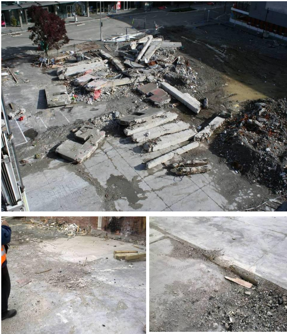
Figure 4 - Ground floor Level 1 slab on grade (clockwise from top) (a) View from snorkel of debris and western portion of Level 1 slab on grade; (b) Slab in northwest corner with column reinforcing protruding; (c) Ramp formed in concrete overlay in front of Line 4 lift core walls.
