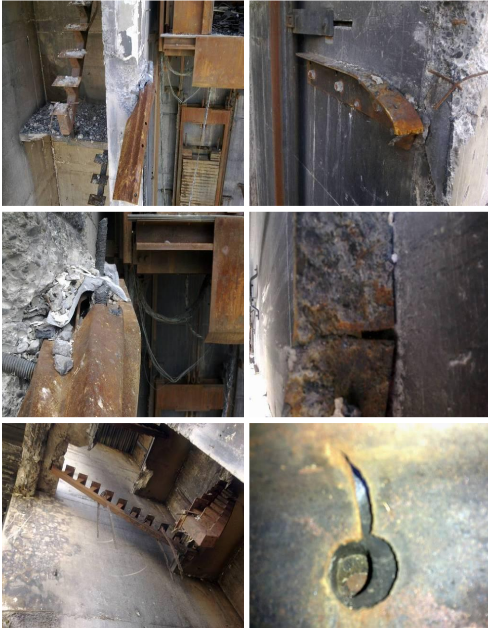
Figure 36 - Level 4 Lift Well Wing Walls Grid D and D/E (anti-clockwise from top left) (a) 150x150x10 L with 51 x 3.2 SHS; 3-M24 threaded rods fixed into wall and 6 –M20 threaded rods 350 mm long fixed into the slab at the profiled metal deck rib with epoxy grout around rod; (b) Three M20 threaded rods remained upright in the Grid D Drag Bar. The 51x3.2 SHS had fractured in bending and tension at the bolt hole adjacent to last bolt into wall; (c) Stair stringer running up to Level 5 fixed rigidly into landings with visible vertical bow (DENG Stair S8 Dwg S31 (Figure 76); (d) Initiation of fracture in the steel angle at the elongated hole without bolt into east wall; (e) Fracture in angle running from corner of angle out towards toe viewed from above; (f) Remnant of 150x75x10 L Drag Bar with 4-M24 threaded rods fixed into grid D/E wall. Angle has fractured in bending and tension two bolts in. End of Drag Bar had been gas cut during de-construction.
