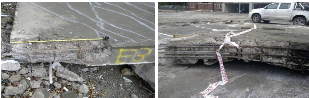
Figure 44 - Locations of H24 reinforcing bar samples (left to right) (a) East end of Line 1 South Wall item E3, one cut from lower 1050 mm of wall; (b) Two lapping bars from lower E3 wall item taken from east end of wall item E4
