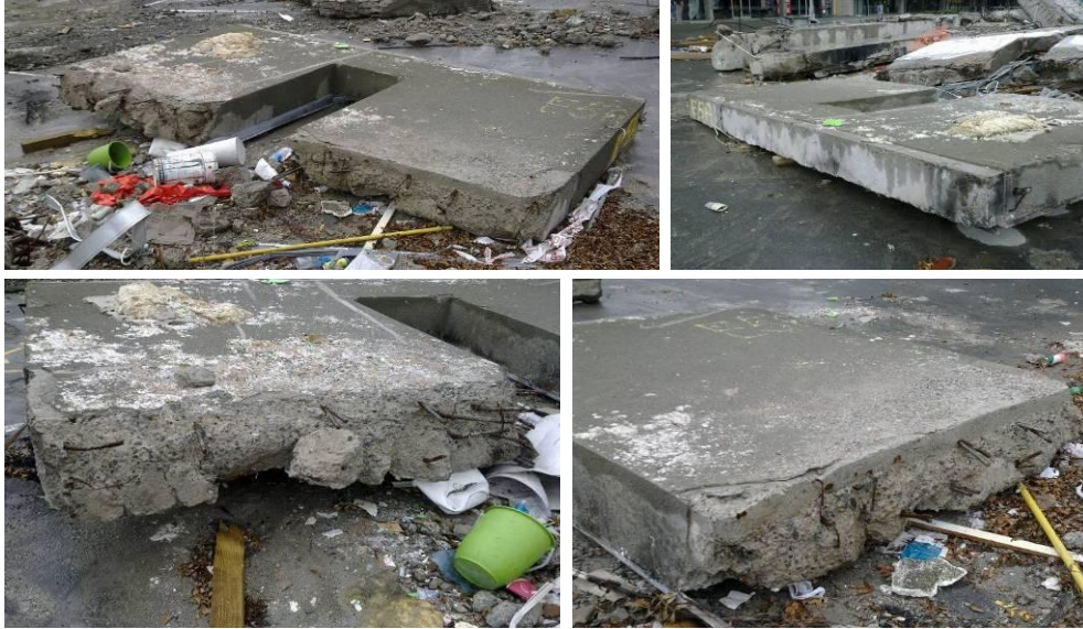
Figure 24 - Line I South Wall Level 6 to Roof (Item E5A) (clockwise from top left) (a) Outer face; (b) Top surface at roof; (c) East pier with saw-cut from de-construction; (d) West pier at construction joint
