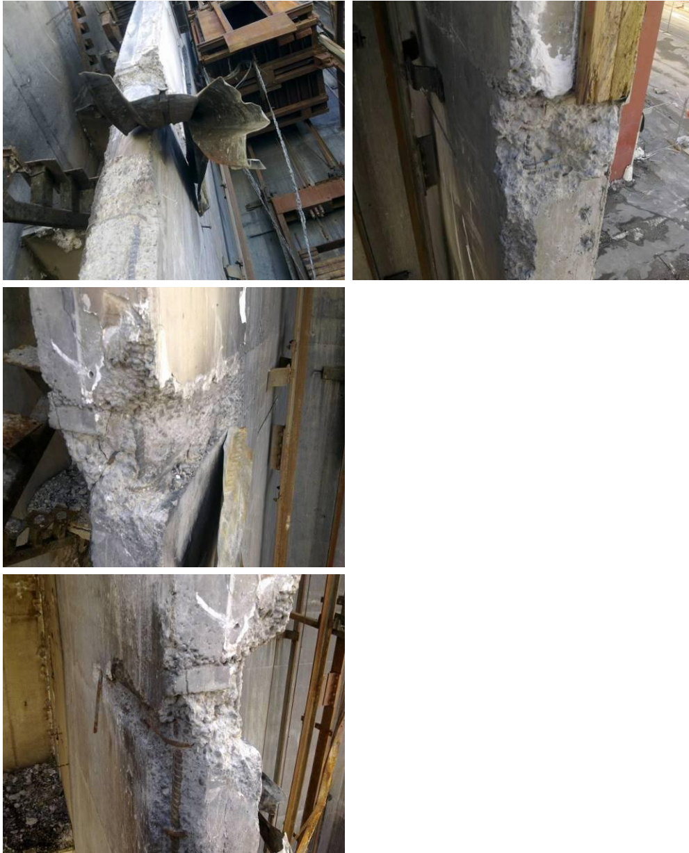
Figure 35 - Level 3 Lift Well Wing Walls Grid D and D/E (anti-clockwise from top left) (a) Profiled metal deck decking side lapped into western Grid D wall, just hanging on; (b) H12 bar necked and fractured at centre of wing wall (indicated by chalk arrow); (c) Concrete cover appeared to have broken away as the slab pulled southwards; (d) Localised spalling of concrete. No reinforcing found connecting end of east wall with slab.
