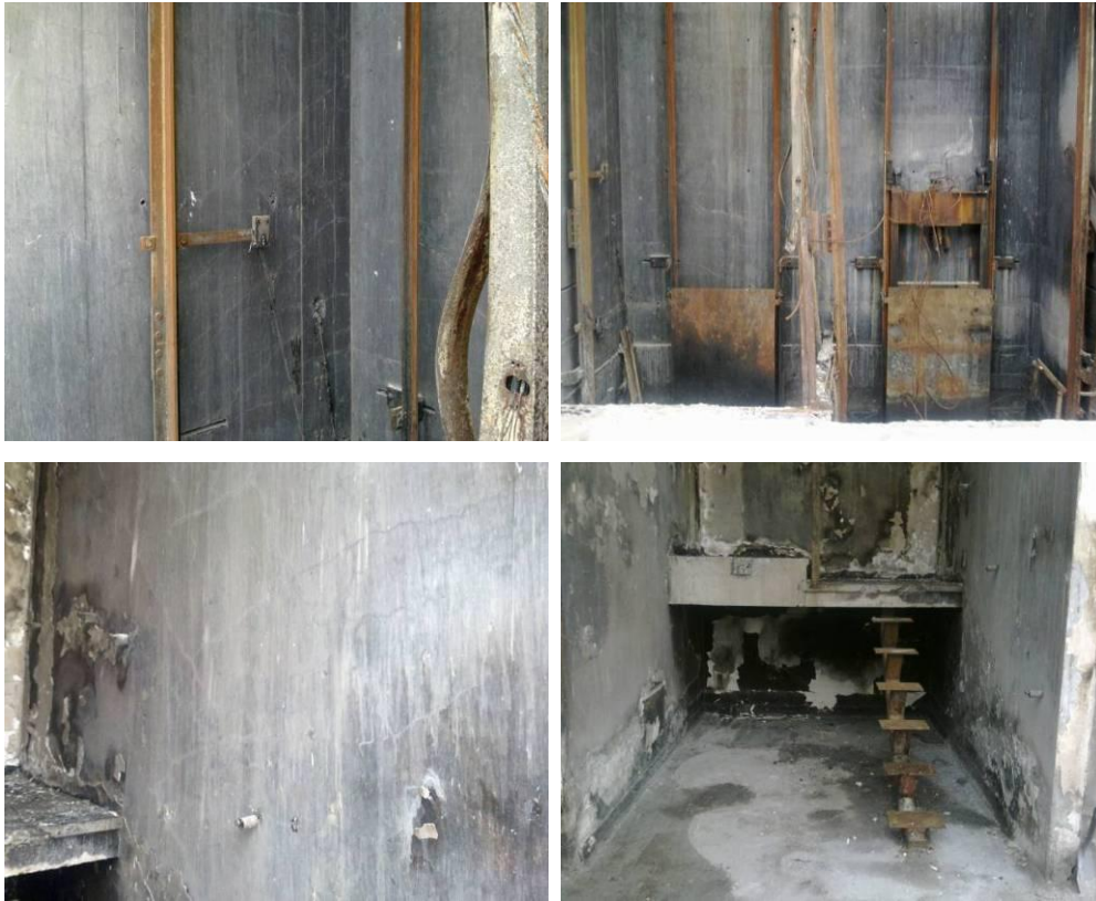
Figure 26 - Lift and Stair well wall cracking Level 1 to Level 2 (clockwise from top left) (a) Lift wall face of Line D wall with fine diagonal shear cracking in both directions; (b) Lift wall face of Line 5 wall with fine diagonal cracking in both directions; (c) Stairwell area with steel stair stringer where concrete cores were extracted; (d) Stair well face of Line D wall with fine diagonal cracking in both directions.
