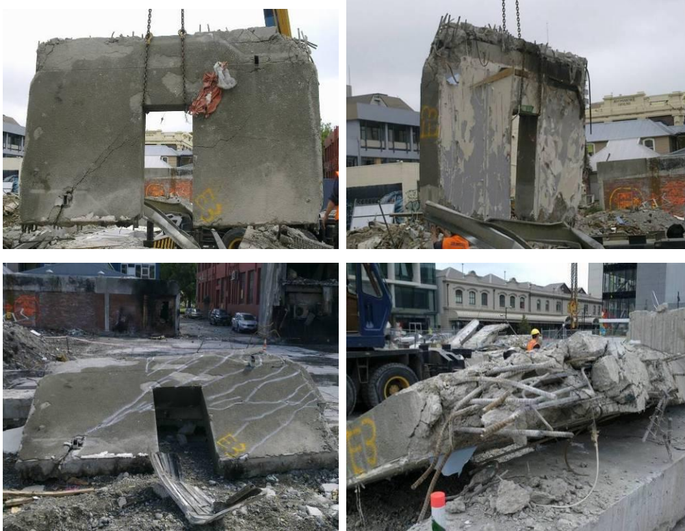
Figure 18 - Line 1 South Wall Level 3 to Level 4 (Item E3) (clockwise from top left) (a) Outer face; (b) Inner face; (c) Damaged top east corner; (d) One way diagonal cracks running from bottom west to top east side marked by paint on outer face.
