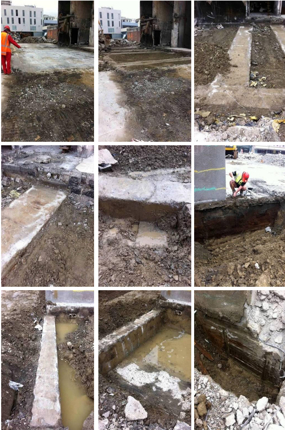
Figure 60 - Foundation Inspection (From left to right in rows from top) (a) P947; (b) P948; (c) P968; (d) P971; (e) P960; (f) P903; (g) P964; (h) P919; (i) P993
