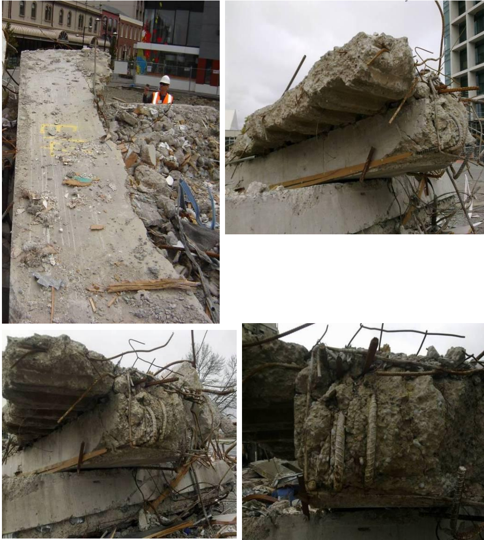
Figure 7 - Pre-cast shell beam (Item E14) from northern face Grid 4, west side of lift core (DENG B23 Dwg S18 (Figure 67)). (clockwise from top left) (a) Top face with slab fracture along edge of shell beam, extending out further at far end adjacent to lift core attachment; (b) to (d) Fractured slab outstand remnant at east end from which slab concrete cores were extracted. The bottom H24 bars from shell beam have been turned back into the concrete infill rather than embedded in shear wall as specified (DENG Detail 5 Dwg S19). Refer also bar imprint on wall at the connection seen in Figure 29 at Level 4 and Figure 30 at Level 3.
