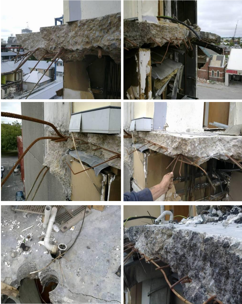
Figure 28 - Line 4 North Core Wall Slab Remnants Level 5 (clockwise from top left) (a) West end with H12 bar ends and mesh at bottom of slab above ribs. It was required on the drawings to be located near the top surface (DENG Dwg S16 (Figure 75)); (b) Looking east. Reinforcing angled down; (c) Slab edge on Grid C west end. Mesh angled down in bottom of slab on top of ribs; (d) Fire charred vertical fractured slab edges adjacent to stairwell. Mesh located low down in slab at top of slab ribs. Edge of mesh sheet with closely spaced parallel wires exposed. Fractured wires can be seen from the lapped mesh below; (e) Cracking in slab running from cored holes; (f) Connection of shell beam to wall with two fractured H24 top bars and two de-bonded top bars. No bottom bars from shell beam embedded in wall (DENG B23 Dwg S18 (Figure 67), Detail 5 S19 (Figure 71)), corresponding to the bent back bottom steel in shell beam Item E23 (Figure 8).
