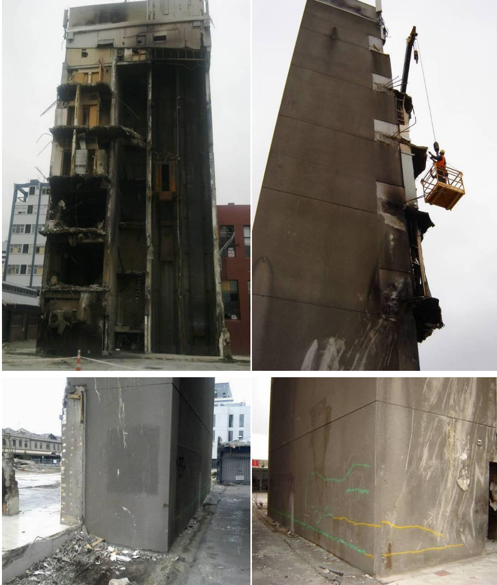
Figure 25 - Line 4 to 5 North Core (DENG Dwg S15 (Figure 65)) (clockwise from top left) (a) South face after site cleared with lift shaft for two cars on right, stair well in middle and amenity rooms on the left; (b) West face; (c) West and north face at Grid C/5 corner Level 1 to 2 with horizontal flexural cracks and construction joint identified by paint; (d) East face with column C18 remnant at far left
