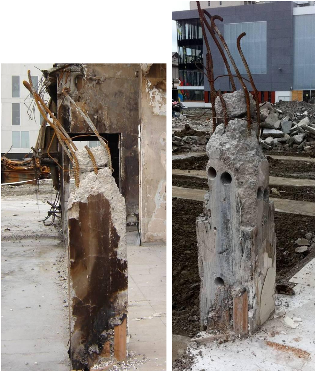
Figure 47 – Locations of concrete cores taken on site for testing on column C18 on Line 4, adjacent to wall D/E
