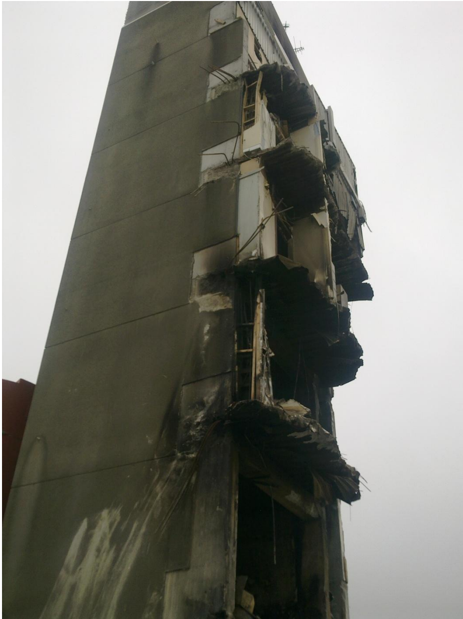
Figure 2 - West face of North Core (Wall Line C) showing the locations where the Line 4 beams had connected into the wall at Levels 3 to 6 without the bottom bars being developed into the wall as specified.
