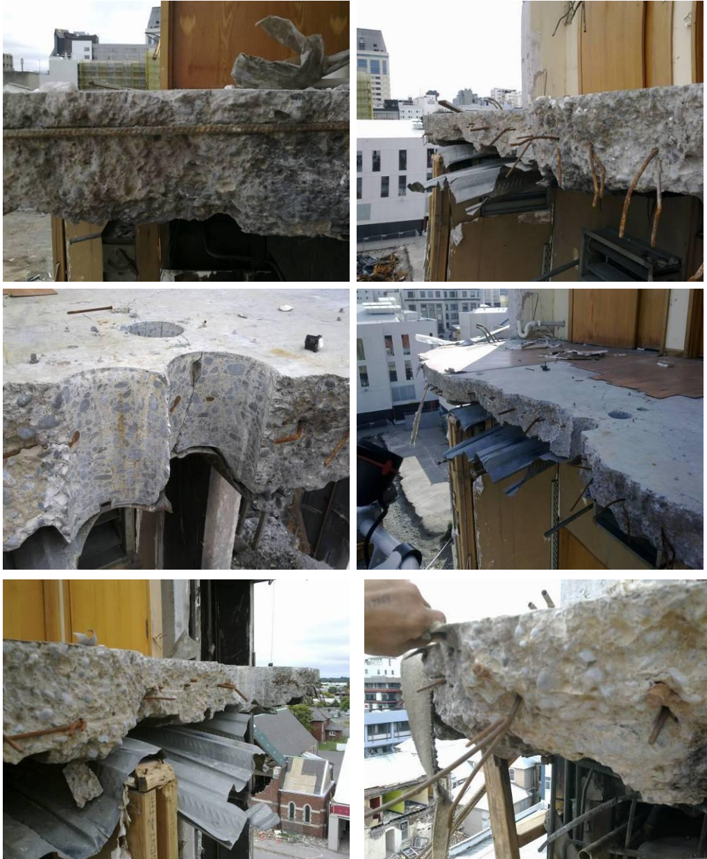
Figure 27 - Line 4 Core Wall Slab Remnant at Level 6 amenity area (clockwise from top left) (a) Slab edge on stairwell wall looking west with H12 saddle bar exposed and ends of mesh below it; (b) Vertical concrete fracture surface with reinforcing mesh fractured; (c) Slab looking west with cores cut in floor for amenities; (d) Fractured mesh angled downwards; (e) Fractured slab edge looking east. Torn metal decking aligned approximately with concrete fracture edge; mesh at varying height within slab; (f) Cores for amenities at fracture edge.
