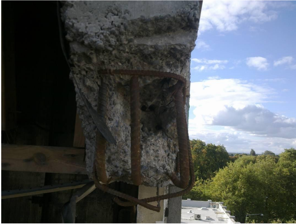
Figure 41 - Lift Well Wing Wall D/E: Column D/E 4 Connection (DENG Dwg S14 (Figure 69); 3 x 20 to 24 mm diameter holes could be seen where reinforcing bars from the column had pulled out. The drawing shows that 4-H20 bars were required to be bent into the wall.
