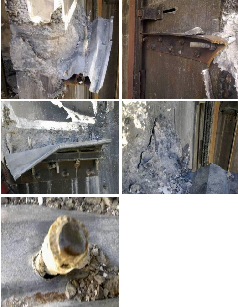
Figure 40 - Level 6 Lift Well Wing Walls Grid D and D/E (anti-clockwise from top left) (a) 150x150x10 L with 51 x 3.2 SHS into west wall on Grid D, similar to Level 5 and 4 Drag Bars; 6-M24 bolts into wall; The remaining 4 -M20 bolts 350 mm long had been fixed into the slab at the profiled metal deck rib with epoxy grout around bolt; These remained vertical and were measured with 110 mm stick-out above the item. The 51 x3.2 SHS has fractured in bending and tension at the bolt hole adjacent to last bolt into wall and the bar had twisted with the slab; (b) Side view of Drag Bar remnant showing deck uplift at end bolt; (c) Top surface of M20 threaded rod with typical smooth diagonal face and grout around rod through slab. (d) End rod with diagonal top surface and slab concrete remains; (e) 150x75x10 L Drag Bar with 7- M24 threaded rods fixed into east wall D/E. End of bar had been gas cut during de-construction.
