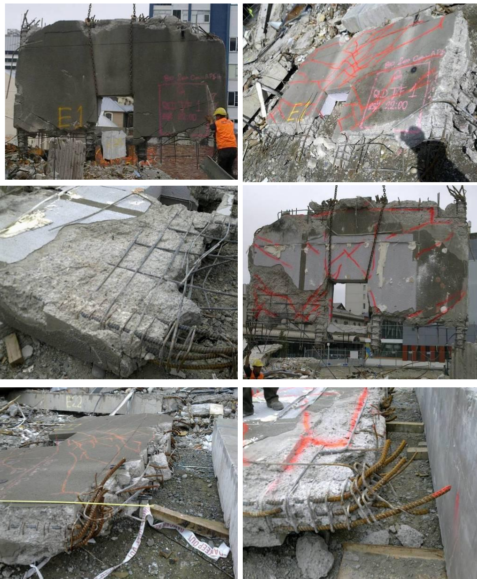
Figure 14 - Line Shear Wall (Item E1) (clockwise from top left) (a) Outer face of wall with lower portion of concrete removed during deconstruction exposing the reinforcing steel; (b) Outer face with cracks highlighted by red paint; (c) Inside face with cracks highlighted by red paint; (d) Top west corner; (e) Top east corner; (f) Inside face of east pier
