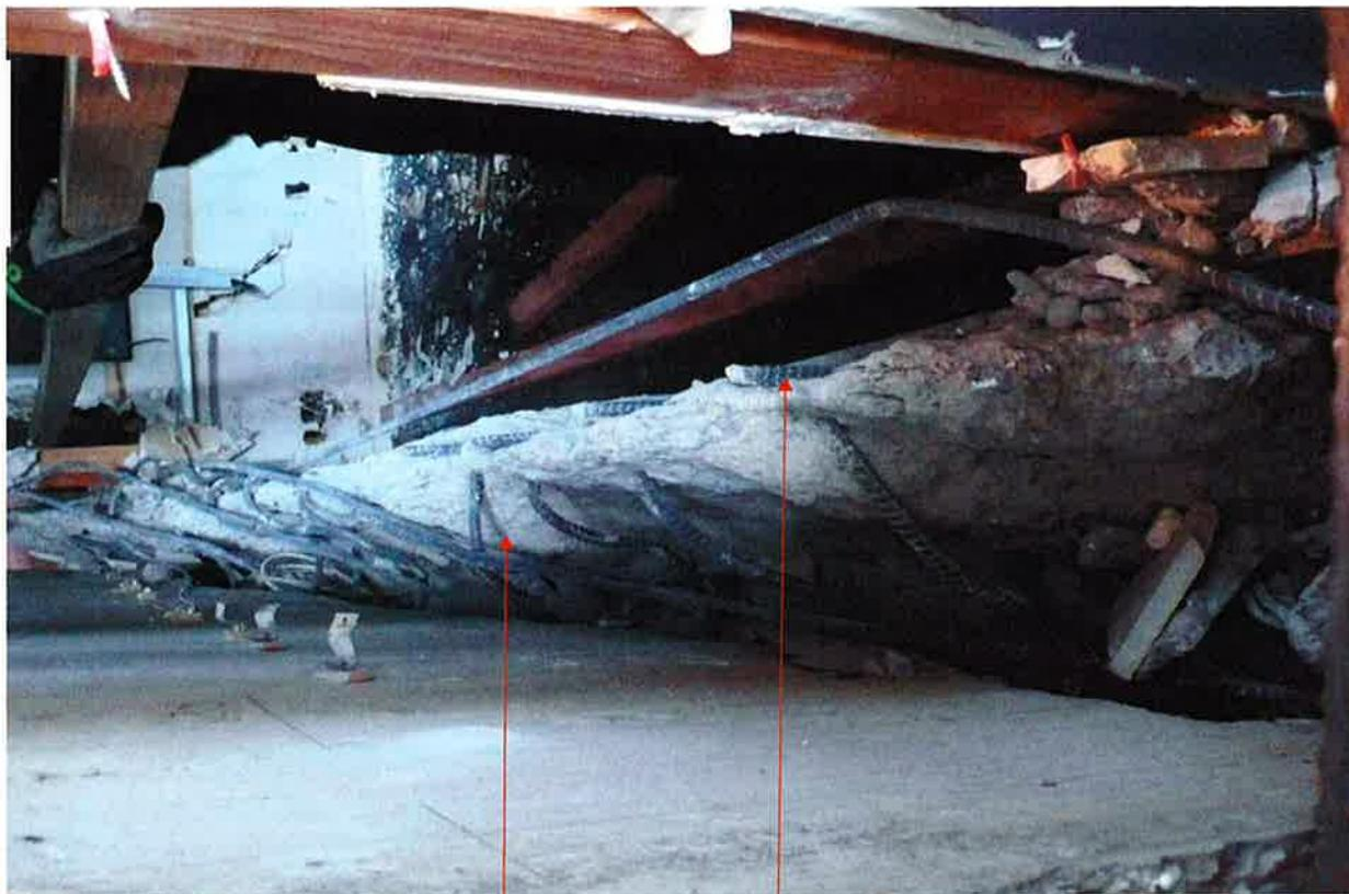
Brittle, transverse failure,
