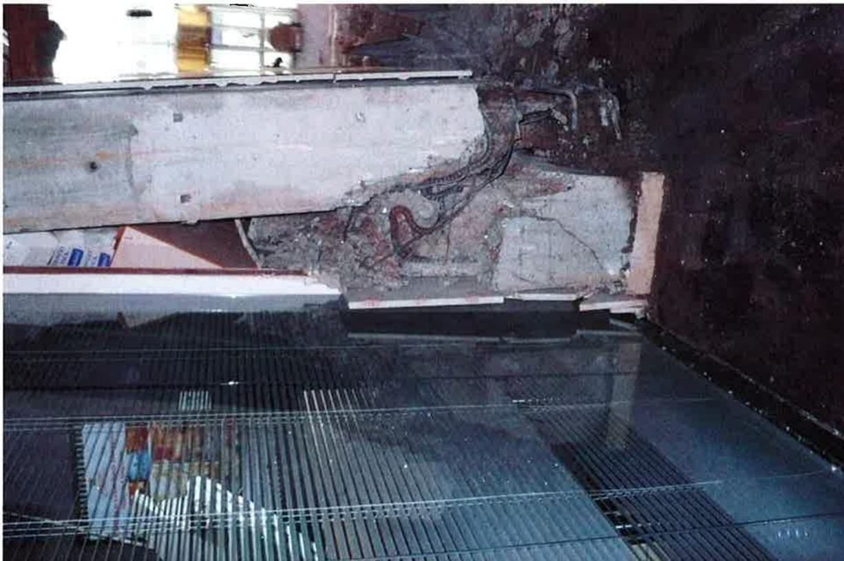
Photo 9 - Shearwall D5-6 Failure - End View
