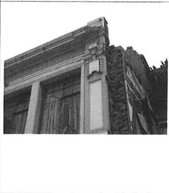
Photo 3 – Wall between 617 & 623 Colombo St
