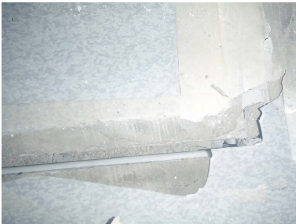
Figure 7.7 : Mortar-Filled Seismic Joint
