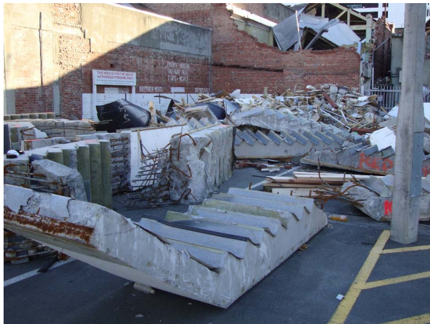
Figure 7.1 : Collapsed Stair Units Removed from Stairwell
