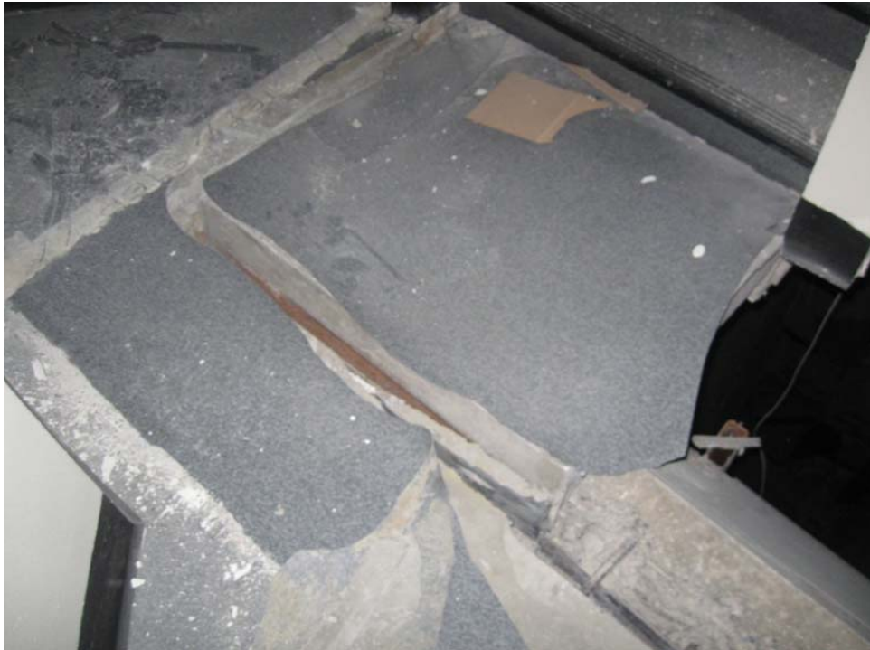
Figure 7.6 : Permanent Displacement at Bottom-Landing Seismic Joint
