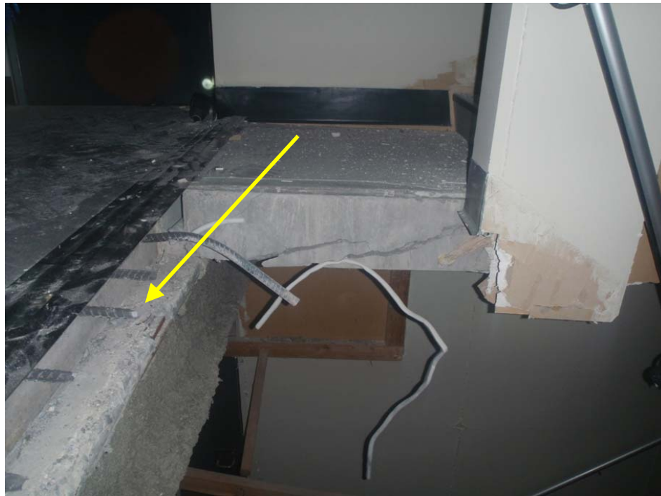
Figure 7.2 : Fractured Top Starter Bars
