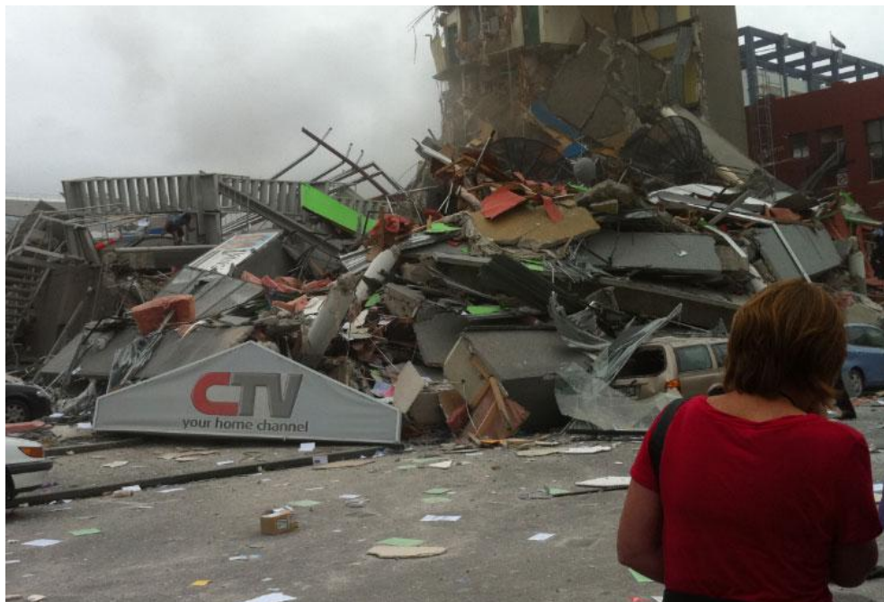
Figure 46 Corner of Cashell and Madras Streets with columns and spandrel panels (msn photo)
