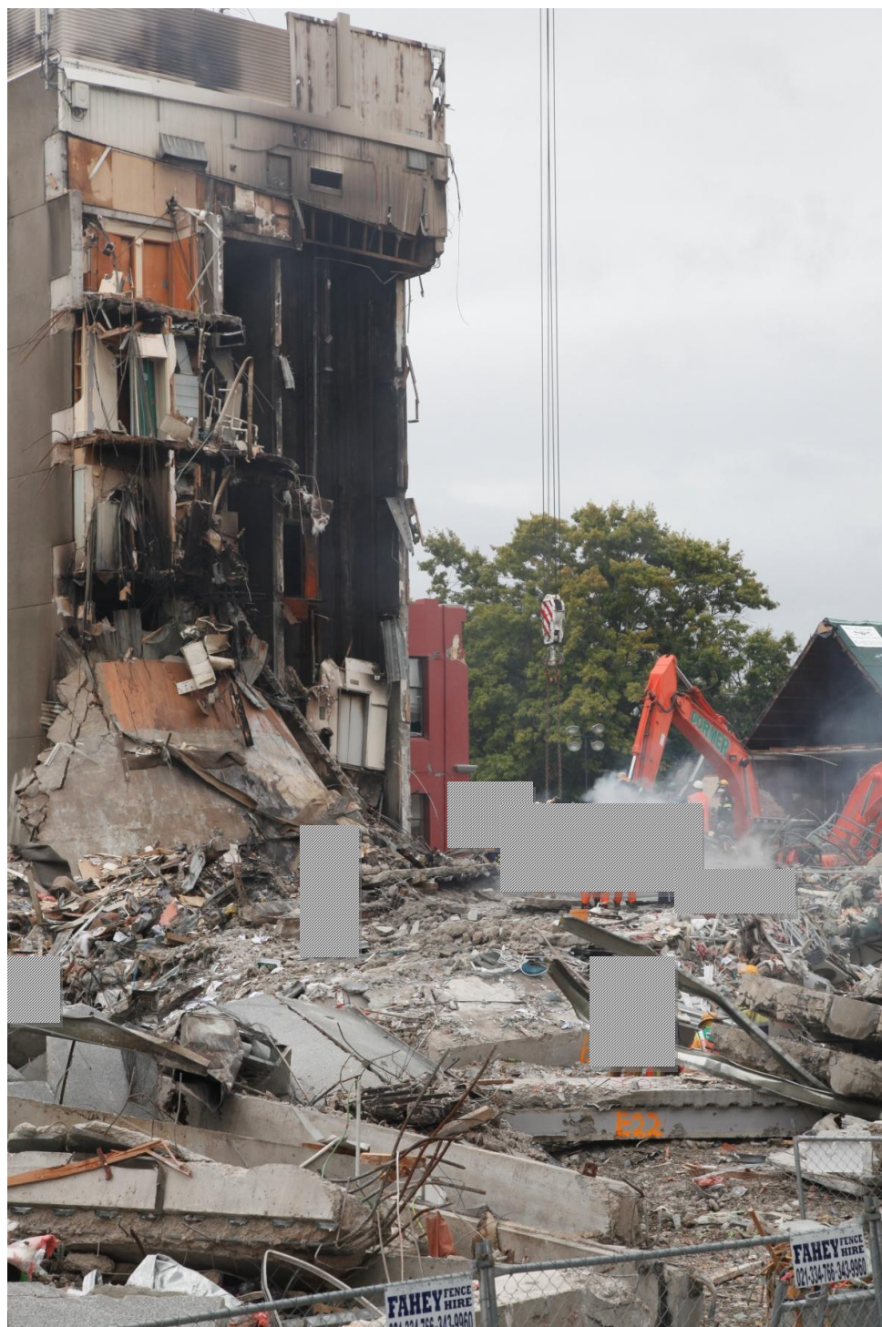
Figure 56 Line I shear wall has been removed.
