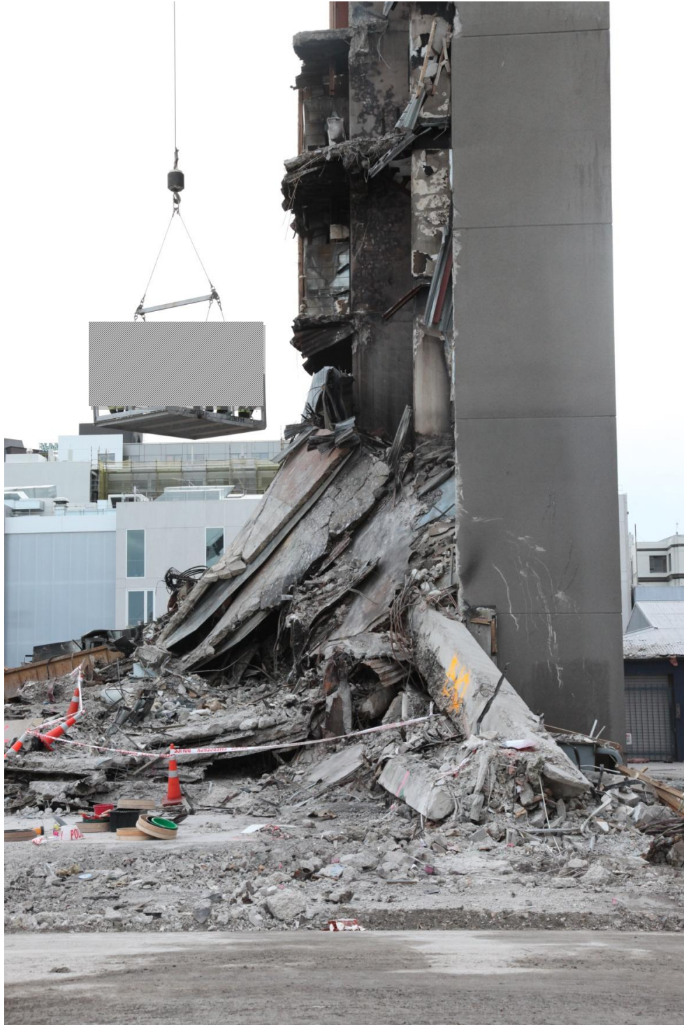
Figure 59 Lift core slabs remaining to be removed.
