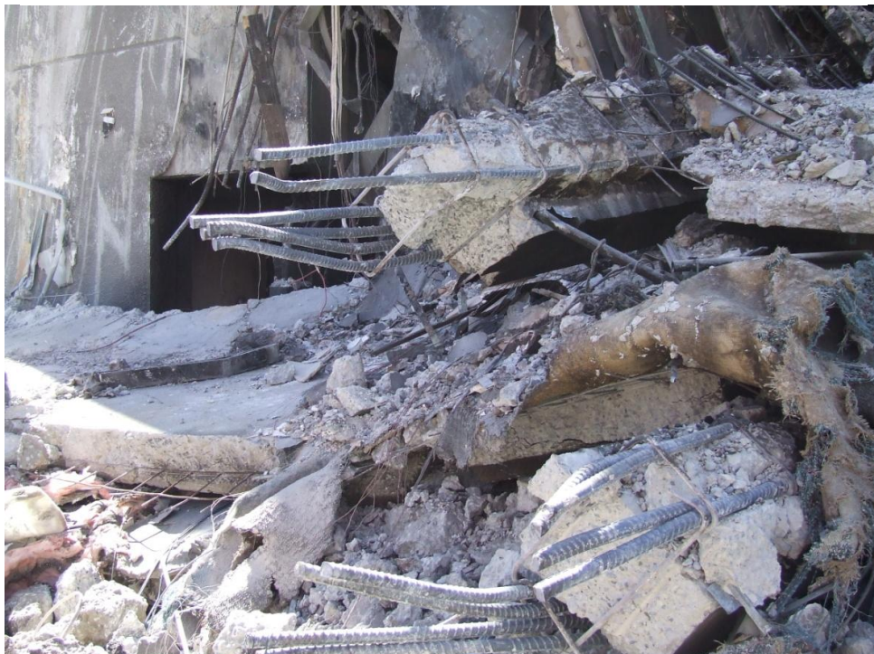
Figure 67 Line 3 beams lying rotated southwards
