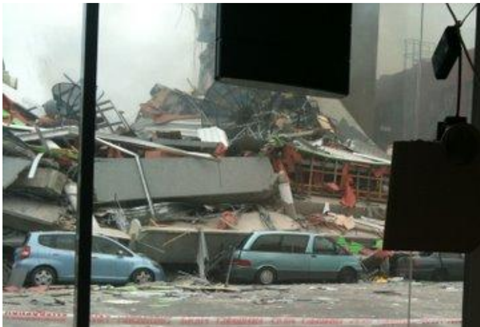
Figure 48 View from across Madras Street with Line 2 column at left and Line 3 column at right
