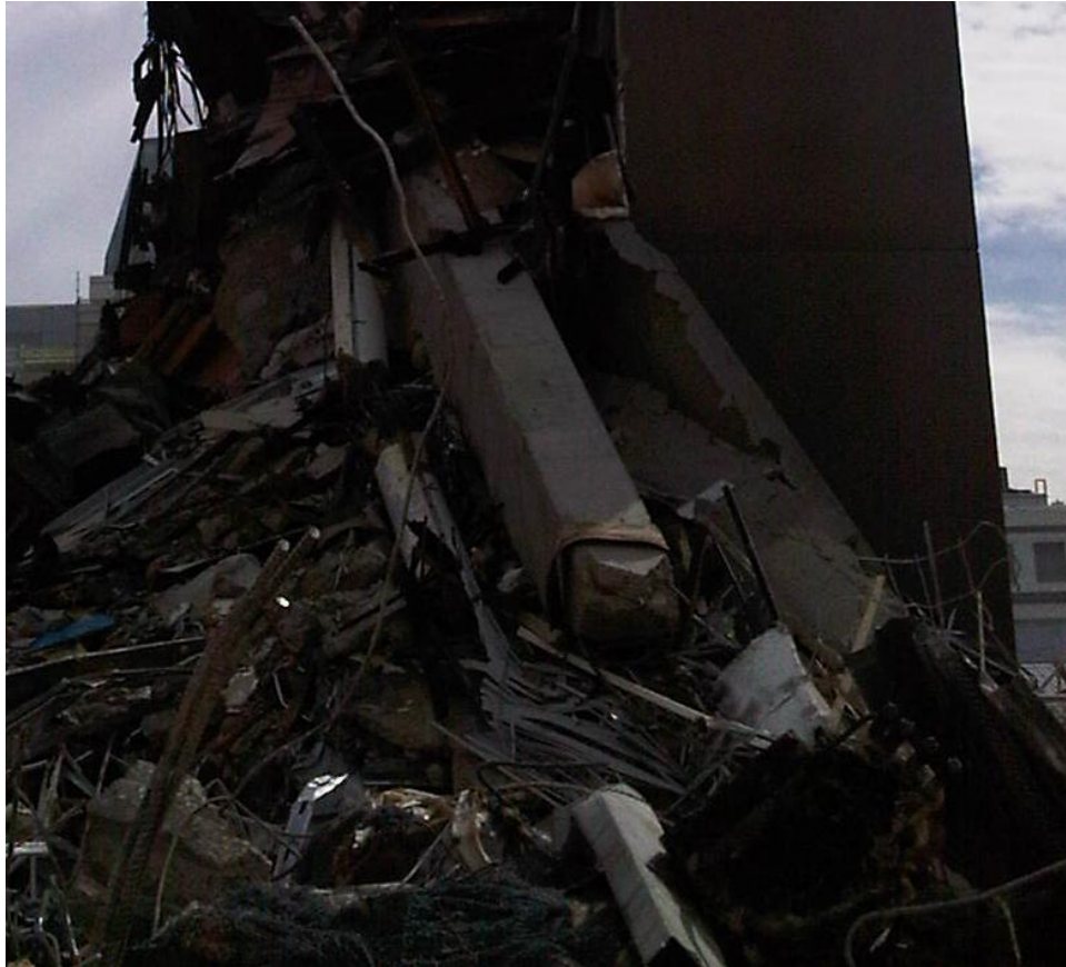
Figure 72 Lift core column C18 remnants among debris
