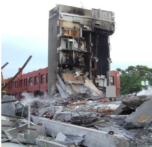
Figure 57 Slabs sloping diagonally from lift core. Line 2 debris still visible
