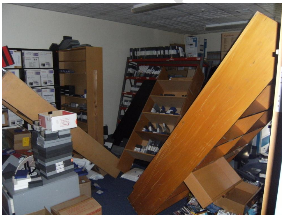
Figure 11 Contents damage on Level 2
