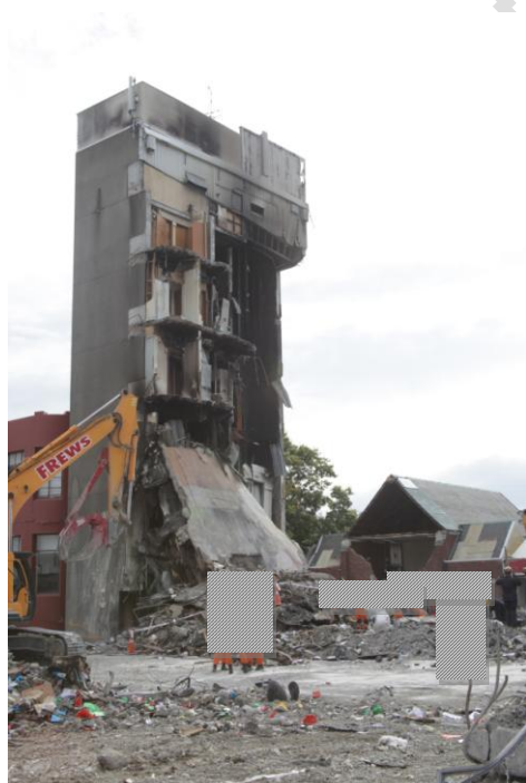
Figure 58 Line 3 and Lift core slab debris remaining
