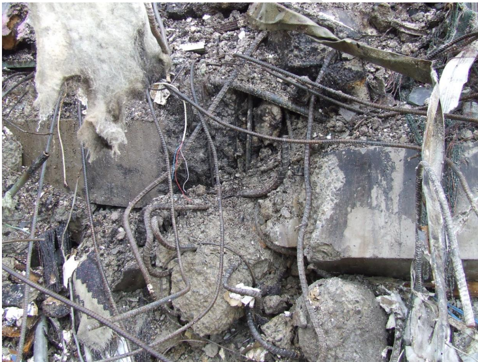
Figure 71 Perimeter columns at beam-column joint with shell beam on right side
