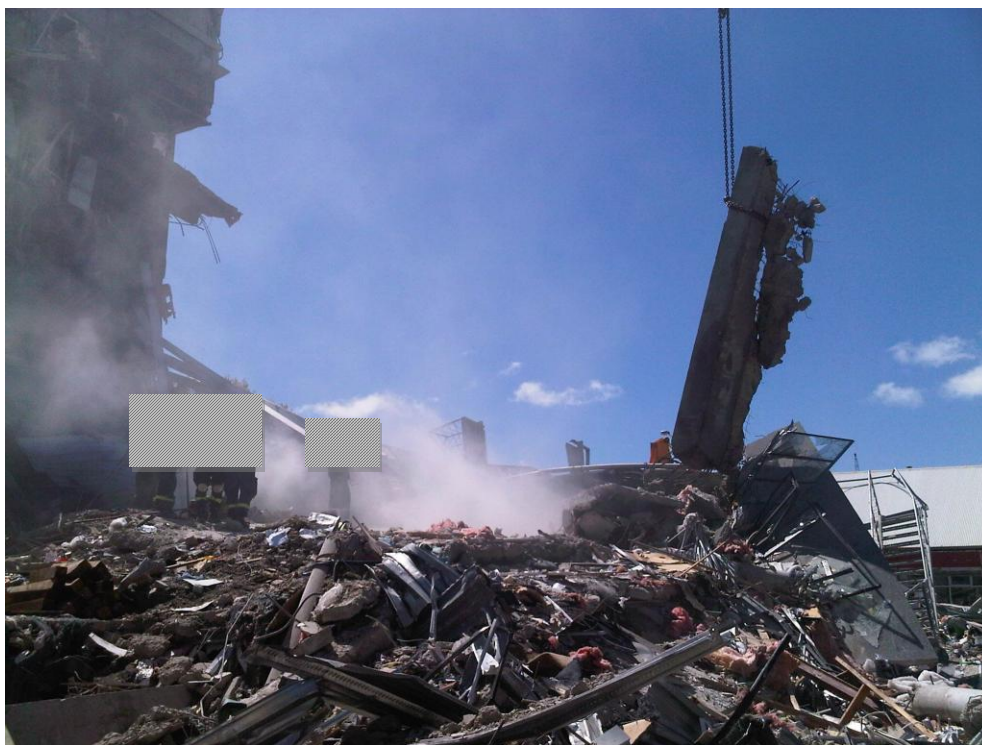
Figure 52 View from southwest corner face Line 1 with pre-cast edge beam being removed and emergency stair on Line 1 shear wall visible.
