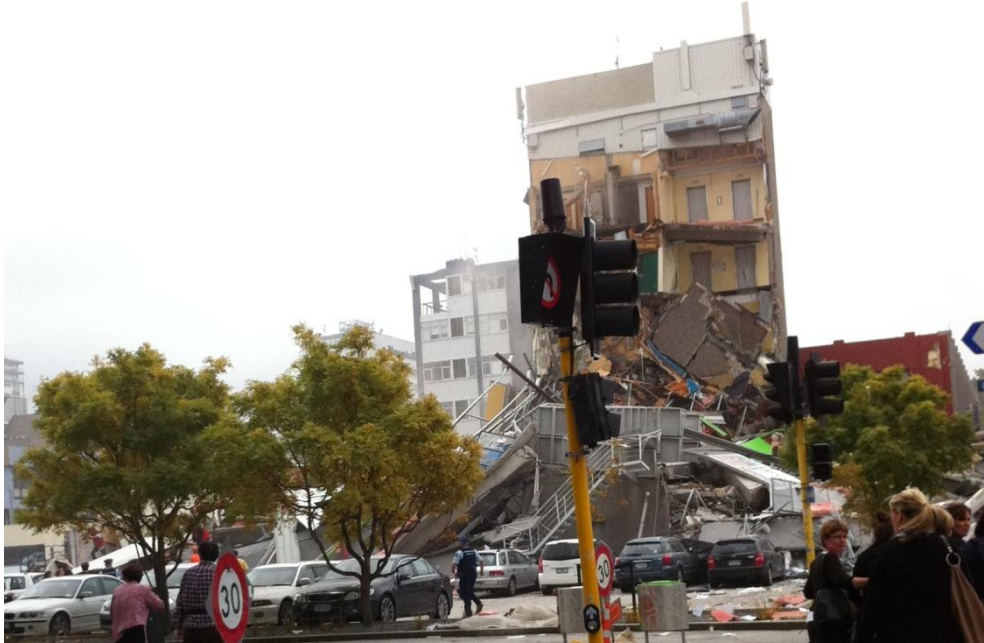
Figure 42 Cashell St face with lift core tower in background prior to fire starting
