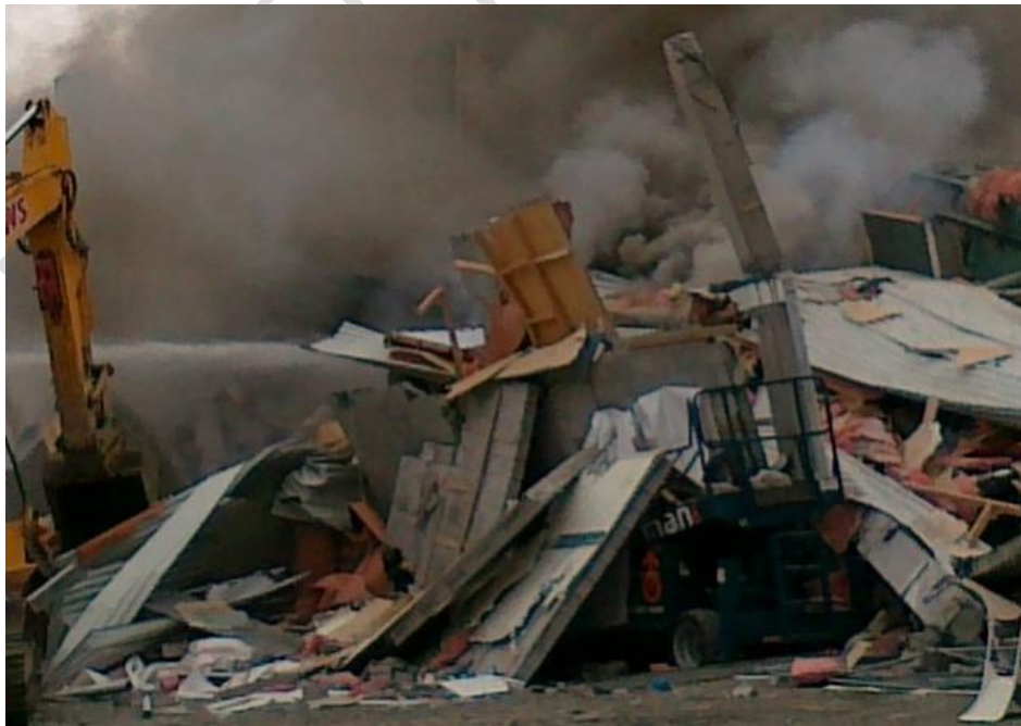
Figure 82 West (Line A) wall at south (Line 1) corner showing collapsed masonry in-fill panels
