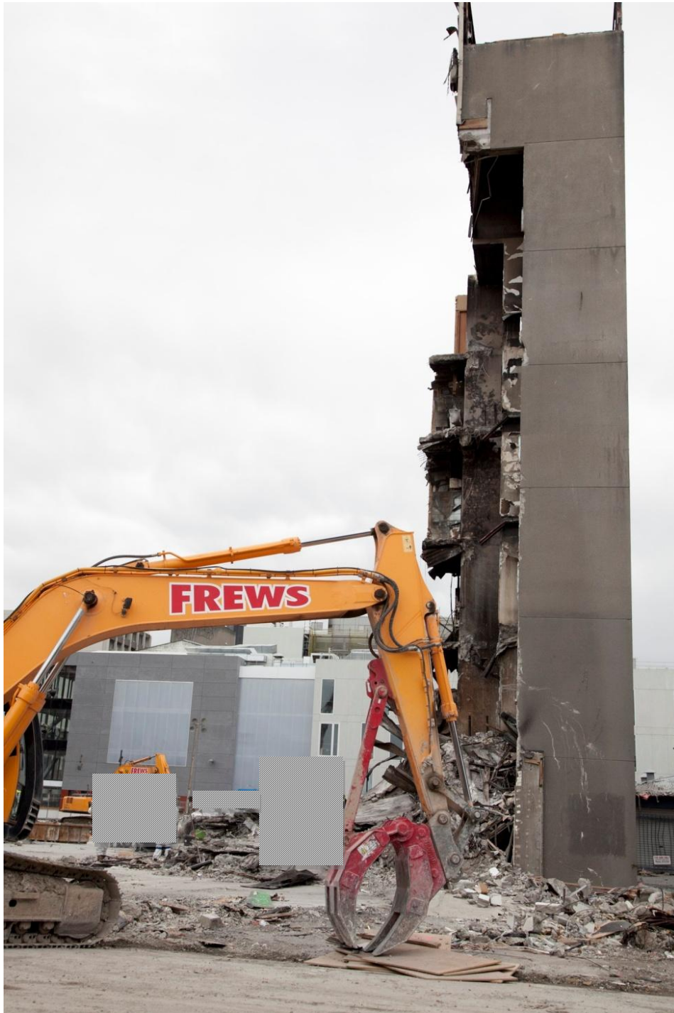
Figure 6 | Lift core slabs removed.
