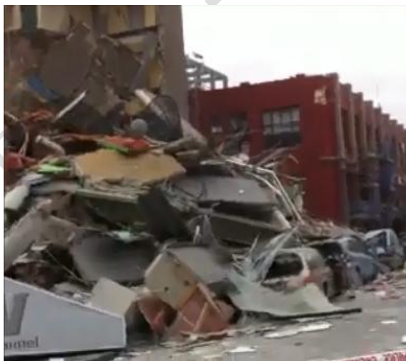
Figure 47 Madras St with precast spandrel panels fallen onto cars
