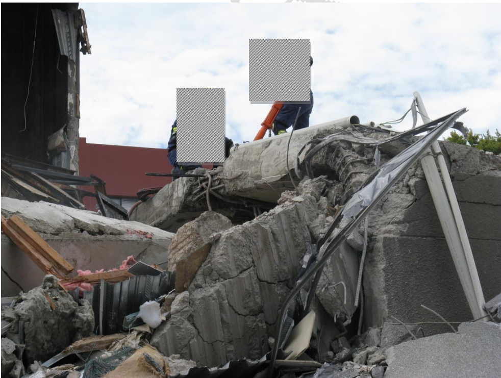
Figure 55 Level 3 portion of Line 1 shear wall being prepared for removal
