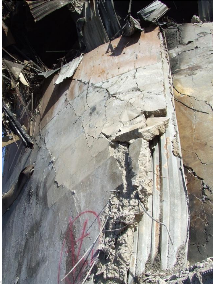
Figure 68 Lift core slab lying diagonally against the core
