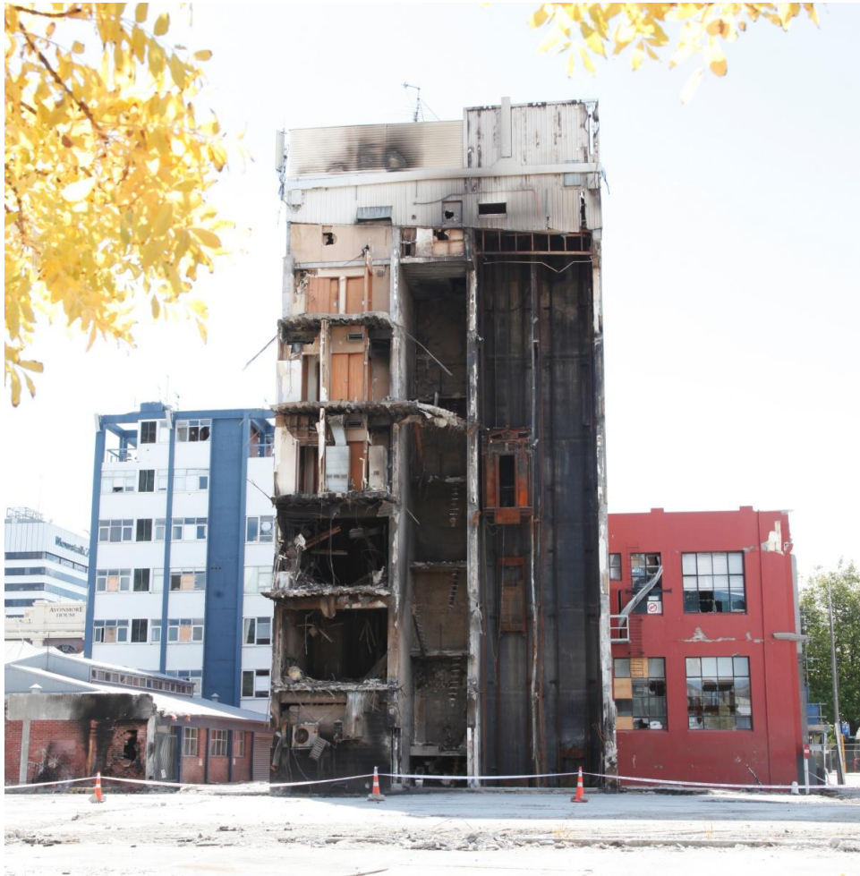
Figure 62 All debris removed leaving the Level 1 slab on grade and remnants of the lift core
