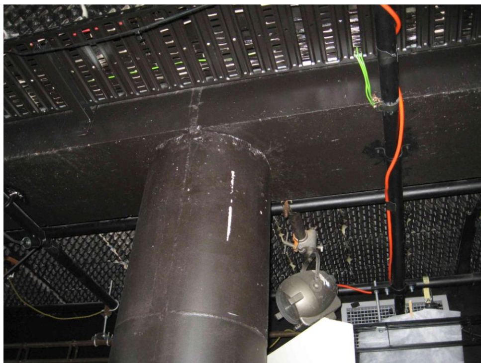
Figure 9 beam column joint on Line 2 or 3 at Level 1
