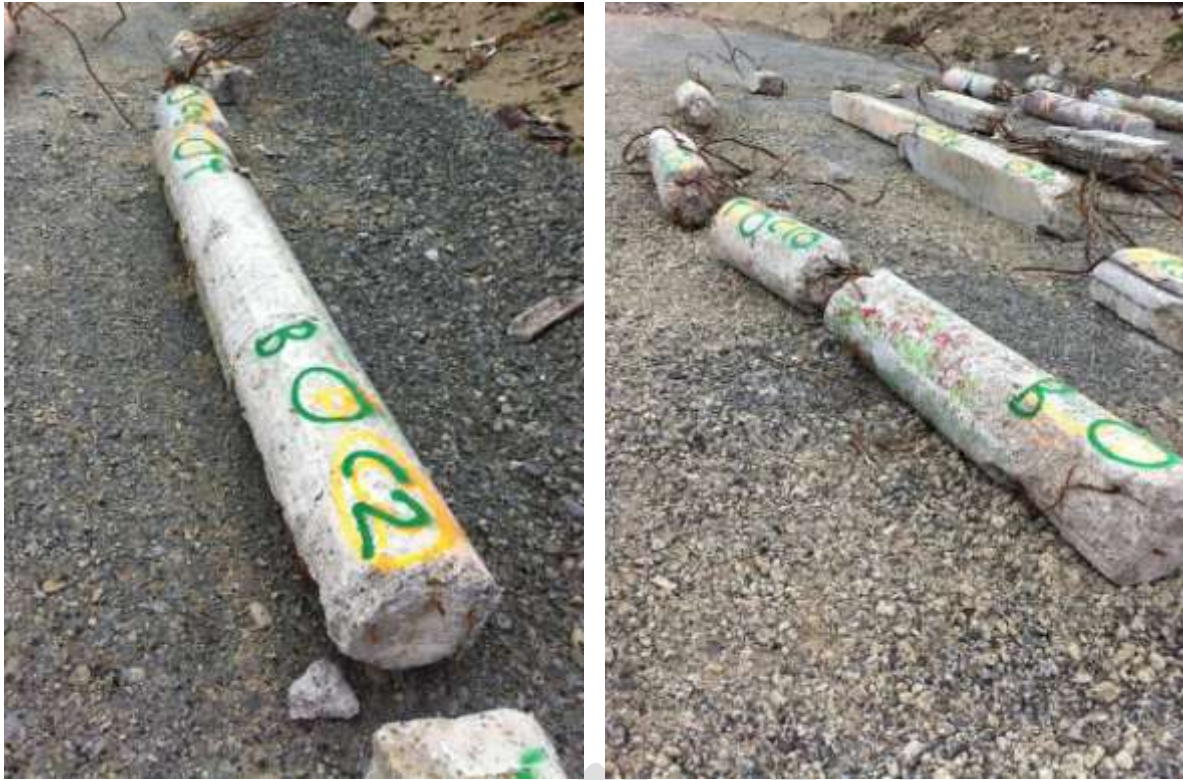
Figure 47 Level 1 Entry 400 mm Diameter Columns (left to right) a) Test item C2, 6-D12 vertical bars fractured at base (DENG Dwg S14 C23); b) Item C10 with down pipe cast in (DENG Dwg S14 C21 or C22)
