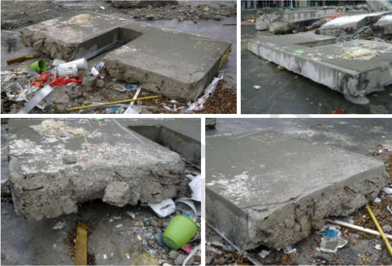
Figure 17 Line 1 Shear Wall Level 6 to Roof (Item E5A) (clockwise from top left) a) Outer face; b) Top surface at roof; c) East pier with saw-cut from de-construction; d) West pier at construction joint
