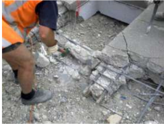
Figure 34 Line 1 Wall Item E1 H16 bars from masonry door infill.
