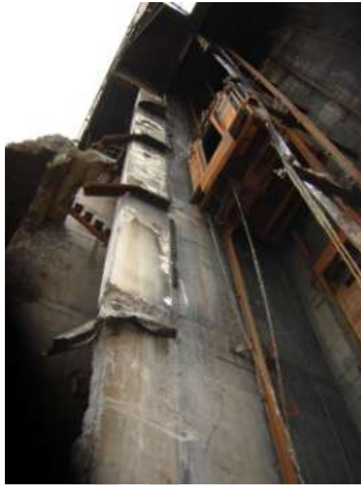
Figure 26 Drag bar connections at Levels 6, 5 and 4 on lift well west wing wall on Grid D. No drag bar at Level 3 or 2 (Figure 25)
